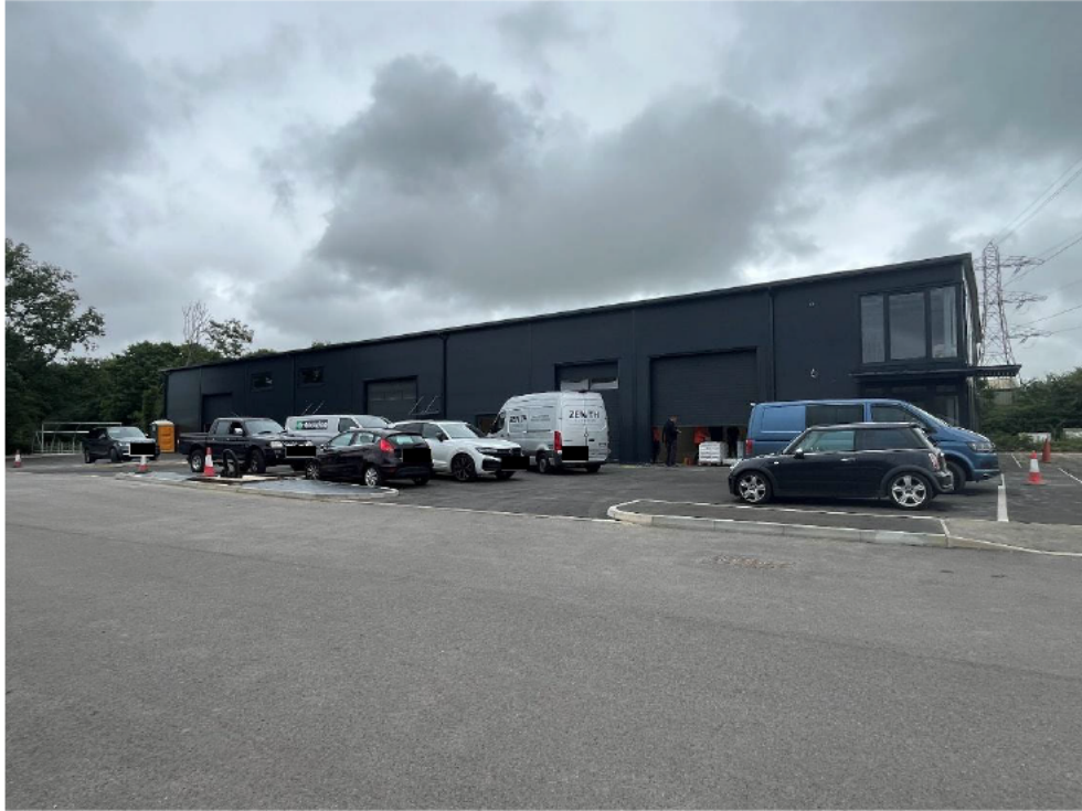
Photo Above: Units 1, 2 and 3 within the Eastern Building
