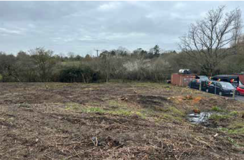
Figure 8 - The cleared site
