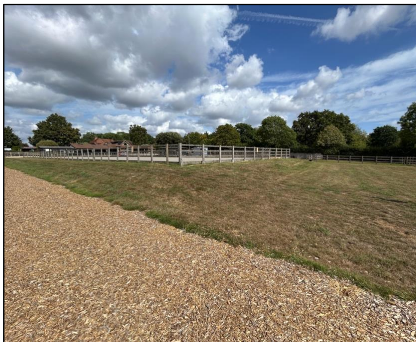
Figure 2: Photograph showing the existing 60 x 20 arena.
