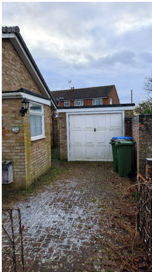
Fig 5: Existing Side elevation showing detached garage and north elevation
