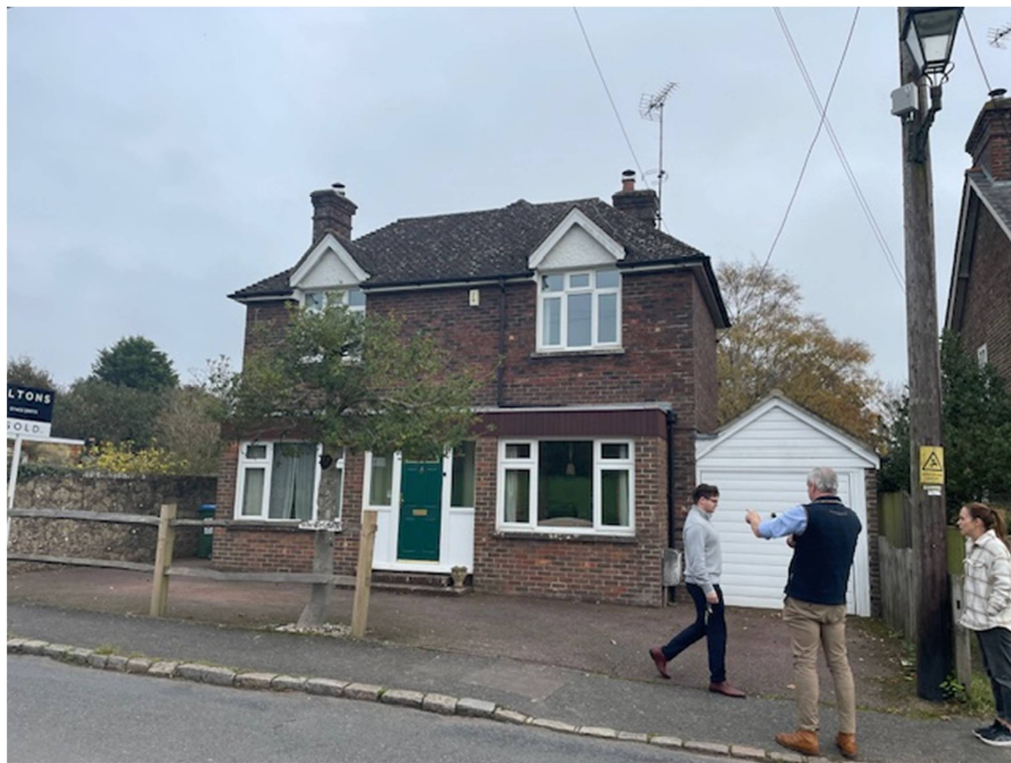
2.9 Photograph of Existing Front Elevation
