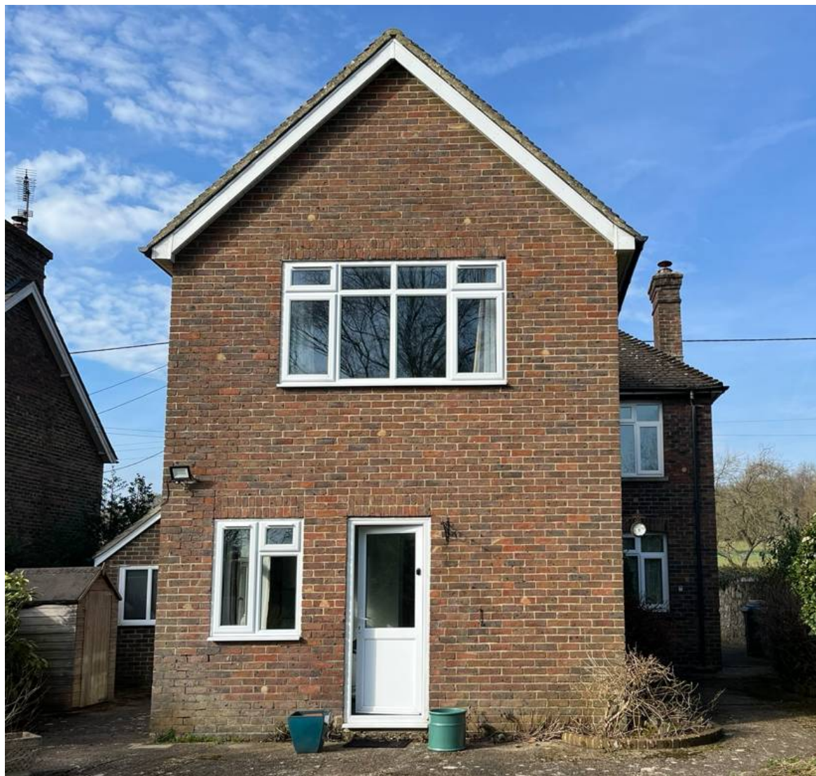
2.10 Photograph of Existing Rear Elevation
