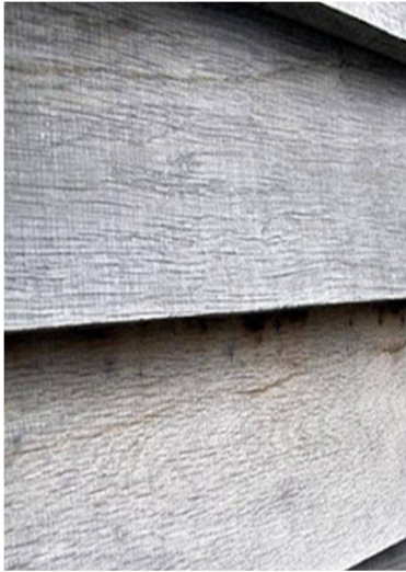
Timber Horizontal Boarding
