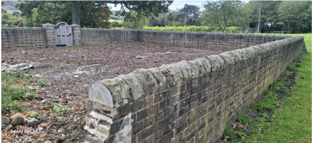
Figure 6 – Close up view of the existing low wall adjacent to the cottages
