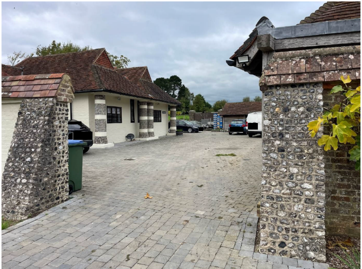
East elevation of listed outbuildings group and showing the butressed courtyard entrance
