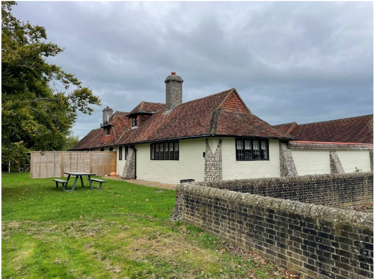
SW corner of Annexe, with the outbuilding group and butressed courtyard wall beyond
