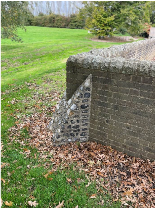
Detail of the existing garden wall (not contemporary with Gerston Hall)
