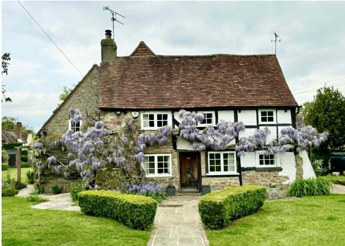
Fig 3: The principal elevation of Cherry Tree Cottage faces east overlooking its main curtilage and drive. It is Grade II listed building and is best appreciated from this aspect, which remains the most original.
