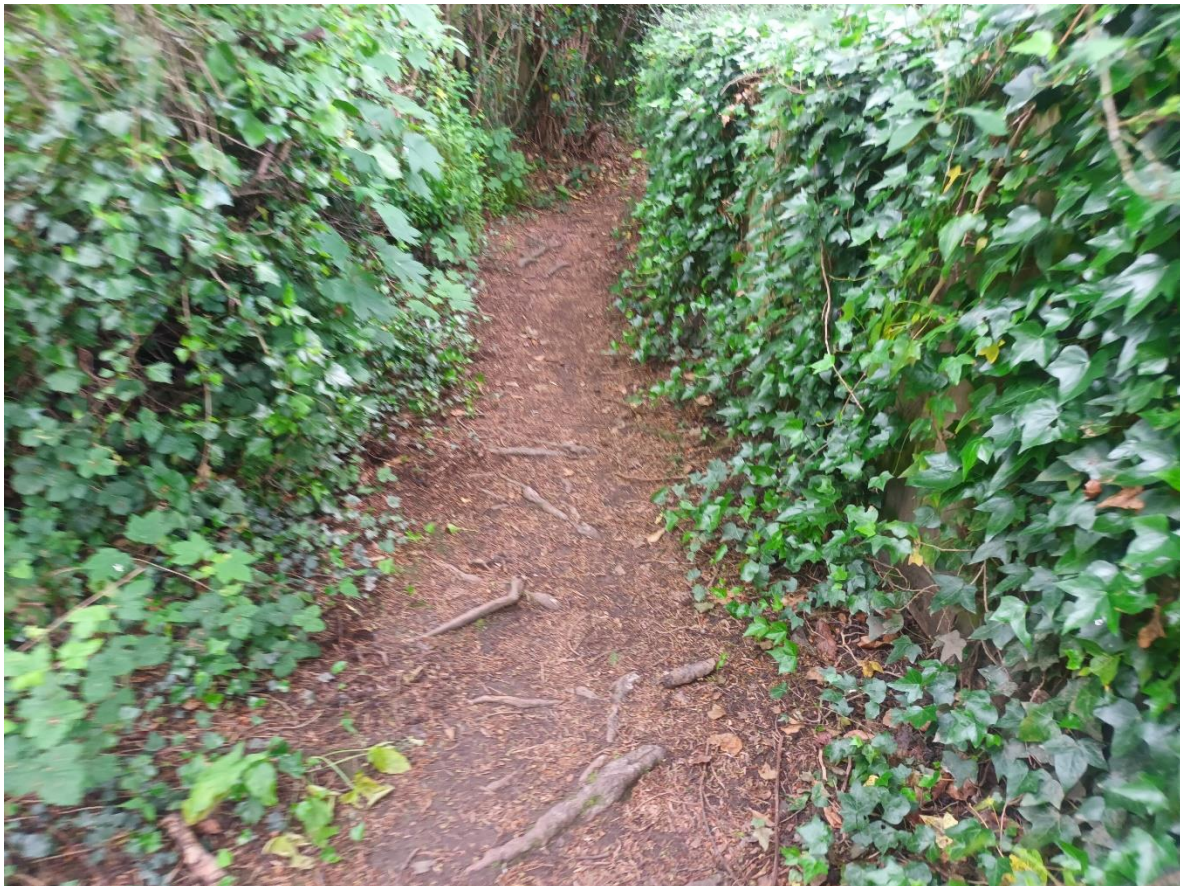
Figure 1 – FP1502 between the northern boundary of the development and Horsham Road showing the influence of tree roots
