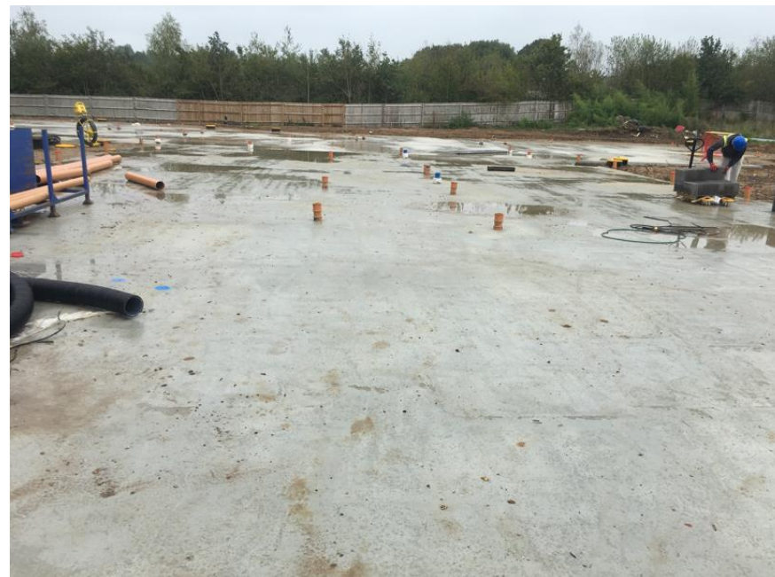
View of the completed ground floor slab covering the location of the former hot spot
