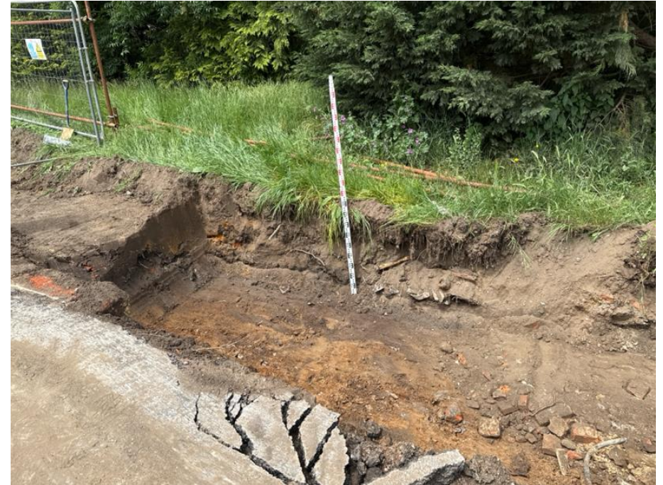
View of the 0.80m deep excavation
