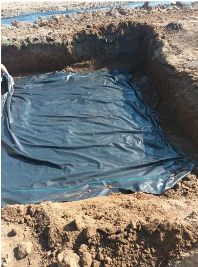
View of the membrane at base of the excavation
