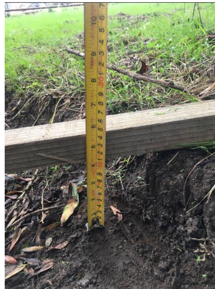
View of the 0.10m deep excavation – northern side
