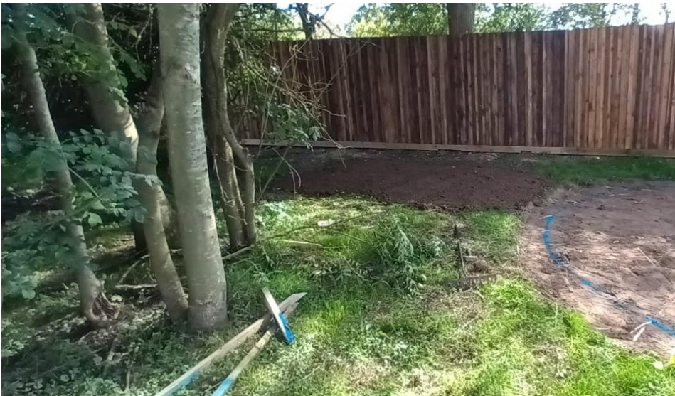
View of the excavation backfilled with Topsoil
