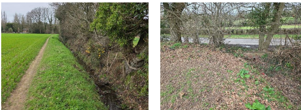
Figure 2-4 On-site ditch running along field boundary (left) and dissused outlet and headwall (right)
