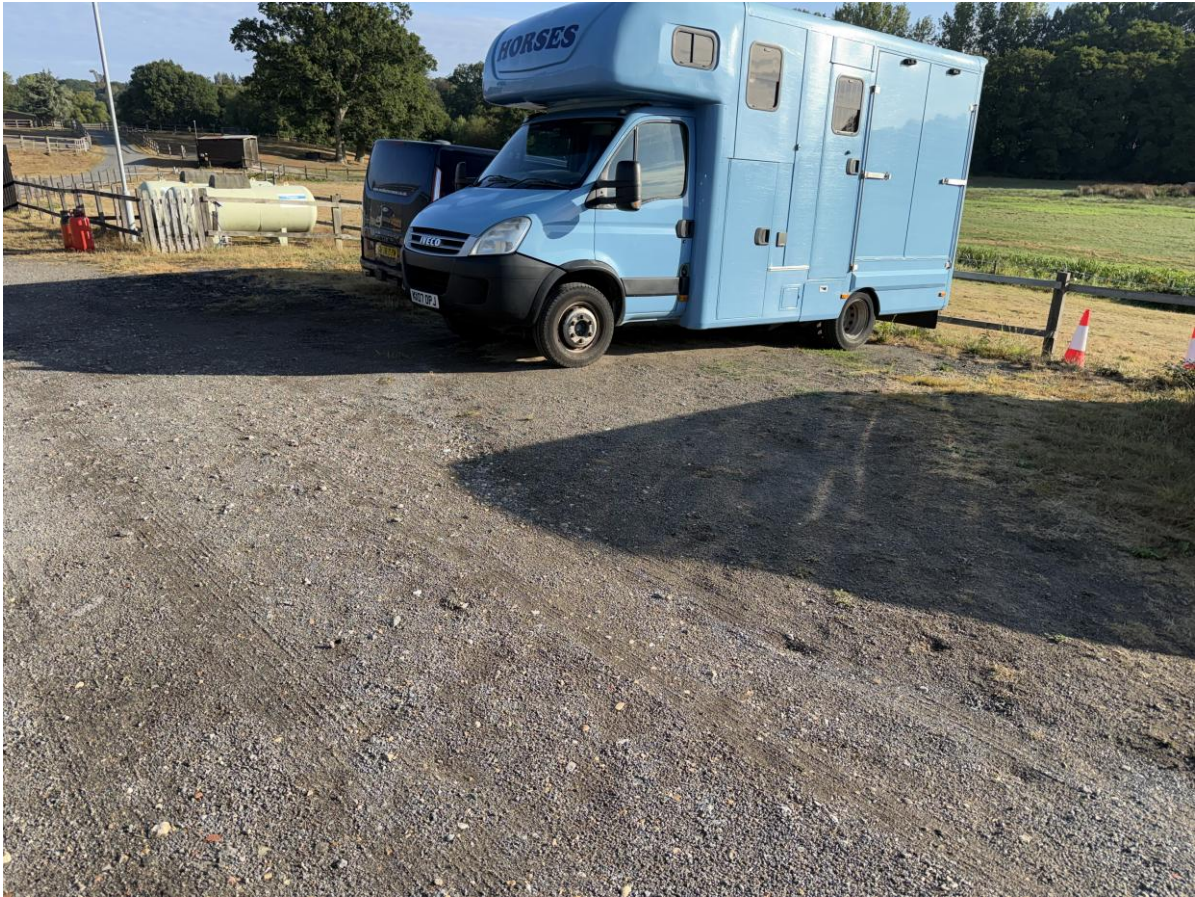
Photo A1. View across the proposed mobile-home area, showing the existing compacted road-planings / aggregate surface and current vehicle parking use.
