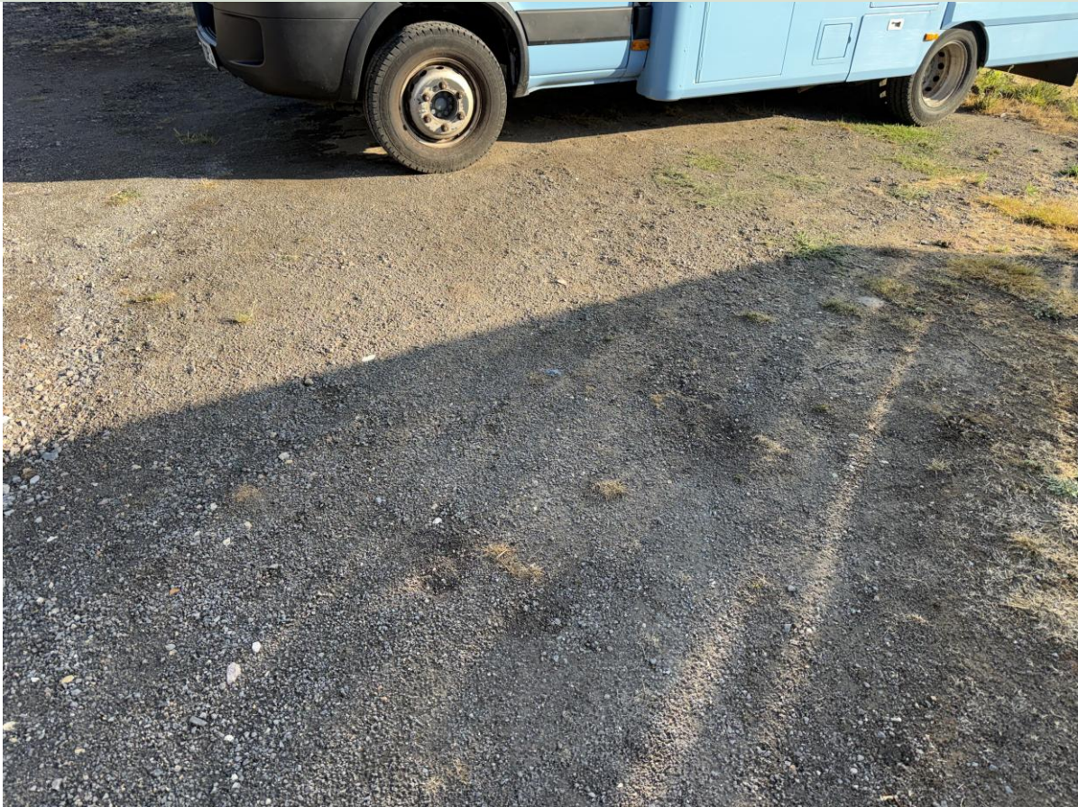
Photo A2. Close view of the road-planings / permeable hardstanding surface, showing sparse and discontinuous vegetation within the trafficked aggregate.
