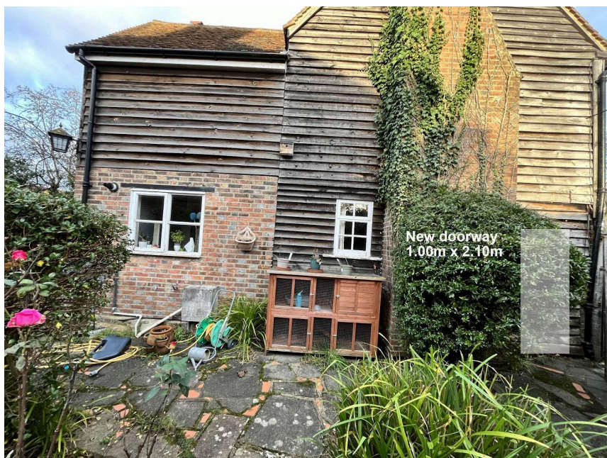
Photograph of external wall where new doorway will be created
