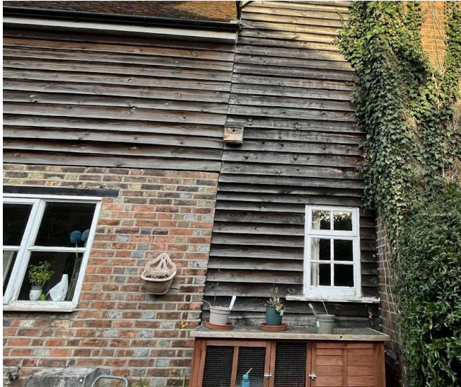
Photo showing how the timber cladding aligns with the front
