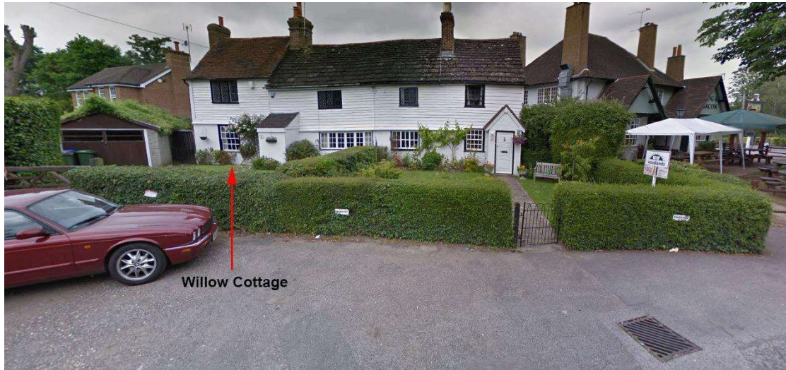
Photograph from North Parade showing the front of Willow Cottage
