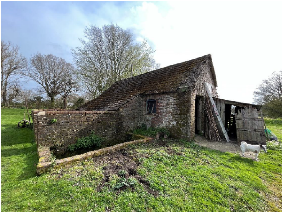
Photo Above: The south and west elevations of the barn and old slurry pit.
