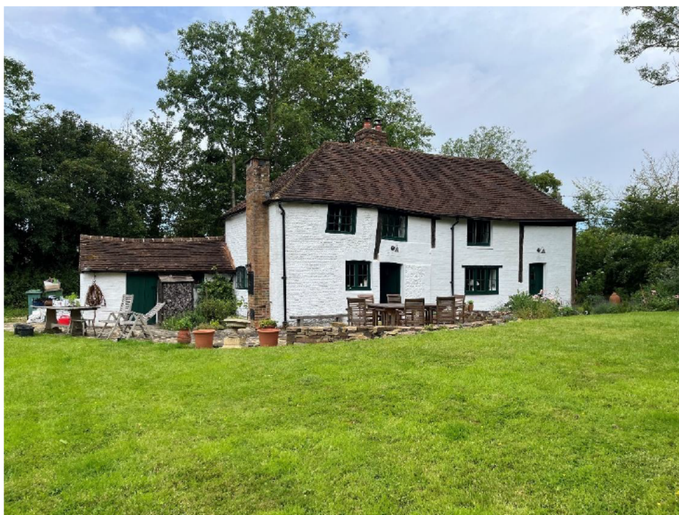
Photo Above: Rear elevation of Harwoods facing the barn.
