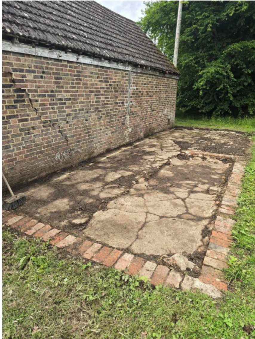
Photo Above: The eastern elevation showing the concrete surface and brick footings.
