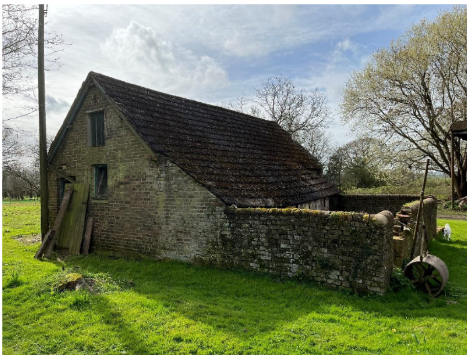
Photo Above: The north and west elevation of the barn (facing the house)
