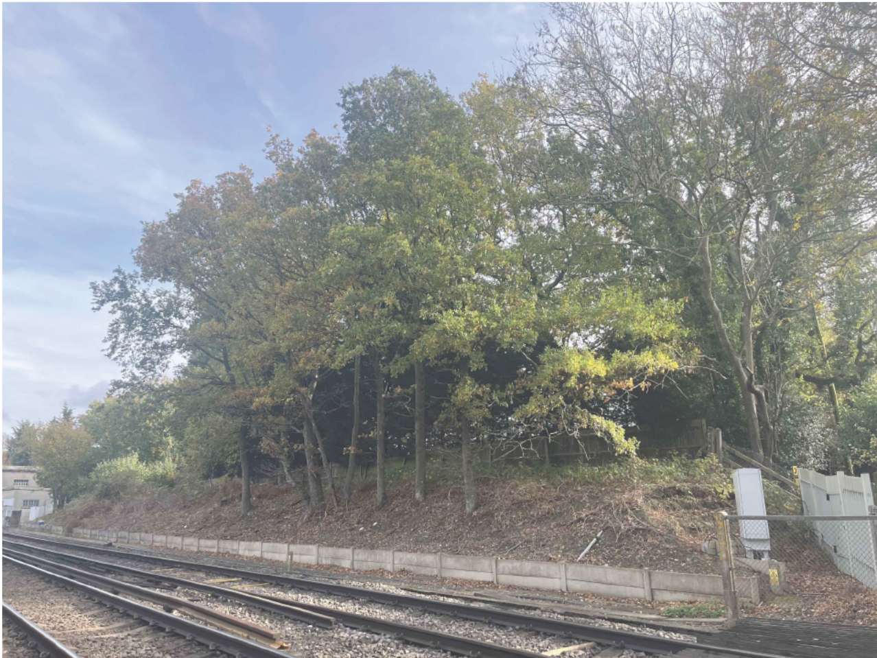
6. VIEW OF RAILWAY BOUNDARY
