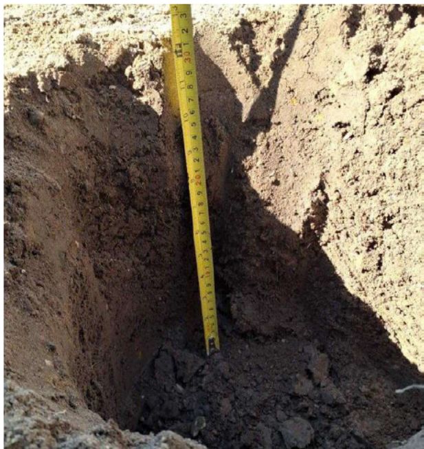
Inspection pit in Plot 14 showing 300mm of topsoil on 30 th September, with further topsoil to be added
