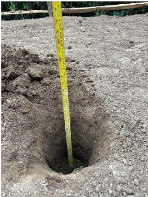
Client provided photograph showing a total 550mm of topsoil on Plot 14, following addition of topsoil
