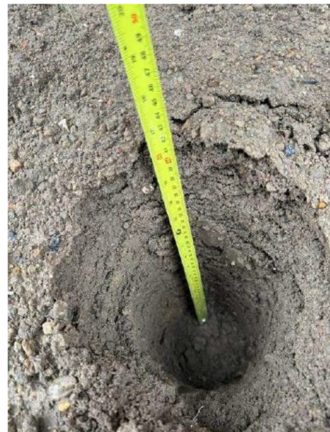
Inspection pit (Apart-1) in Apartment block area on 28 th October 2025 showing 450mm of Topsoil
