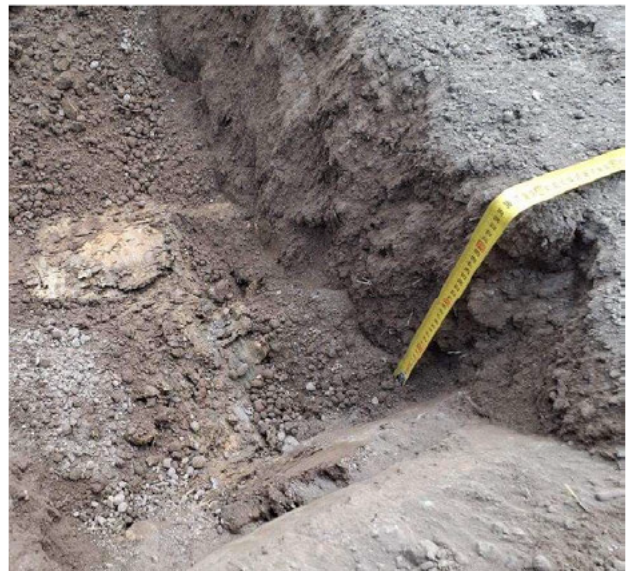
Inspection Pit in Plot 11 showing 350mm of Topsoil and Formation Soils at the Base
