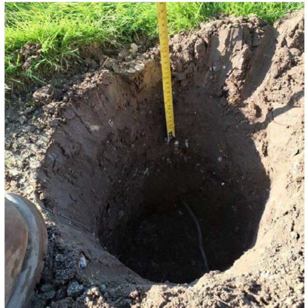
Inspection pit POSHP1 in Central Area on 30 th September 2025 showing an additional 200mm of topsoil placed over the area
