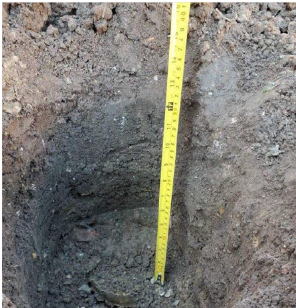
Inspection Pit in Plot 5 showing 350mm of Topsoil and Formation Soils Beneath
