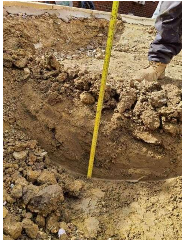
Pit excavated into formation level of Plot 7
