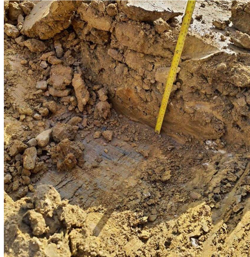
Inspection pit excavated 350mm into the formation level
