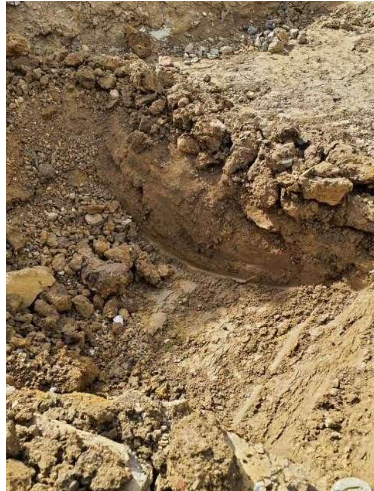
Pit excavated into formation level of Plot 7
