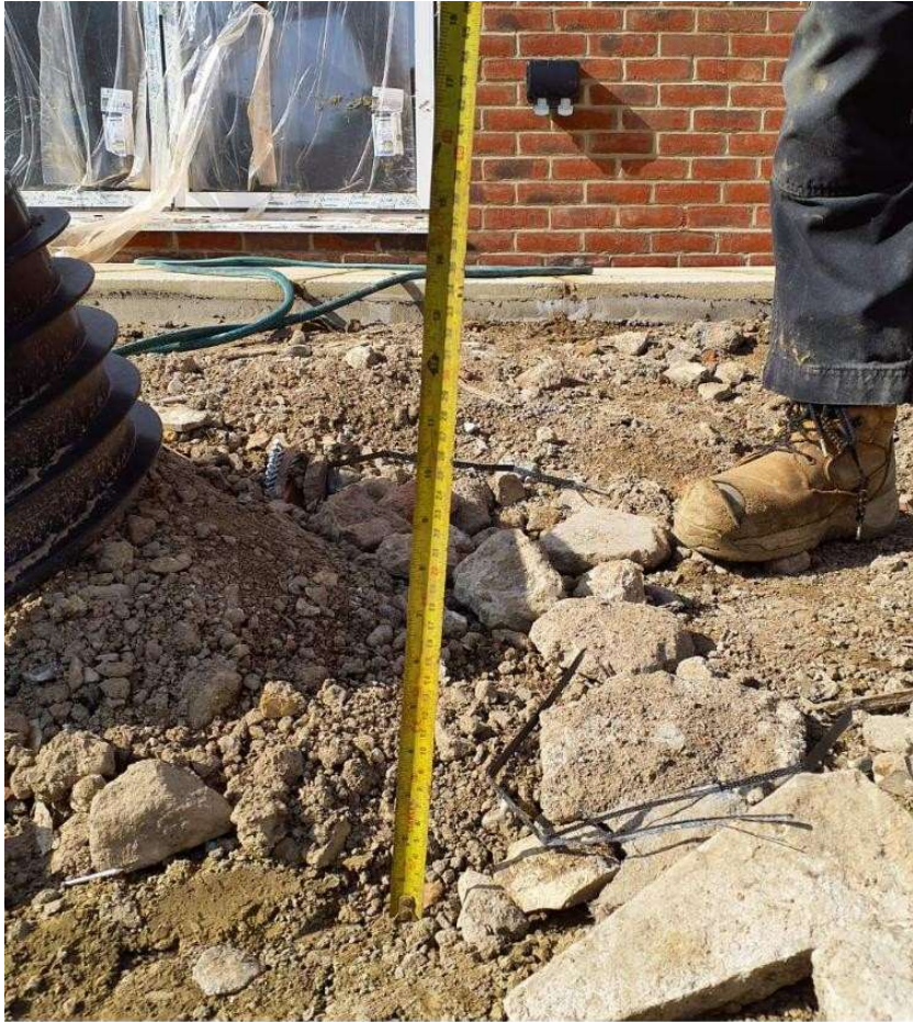
Tape measure showing reduction in formation level by 350mm
