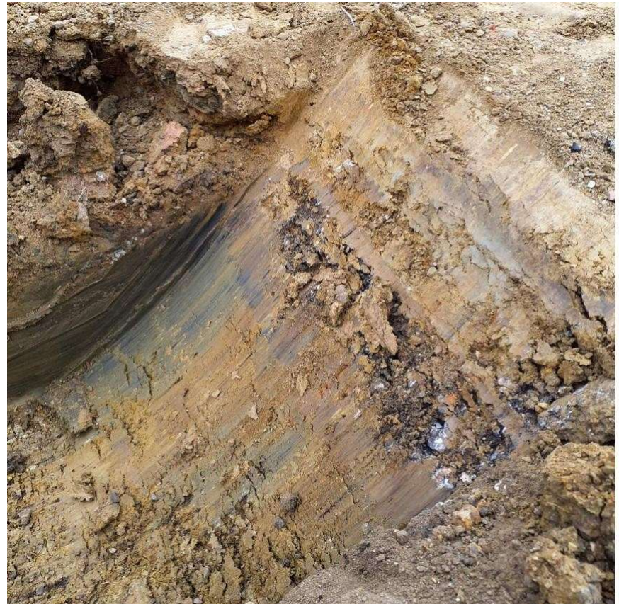
Inspection pit excavated into the formation level indicating made ground was present in the formation level soils
