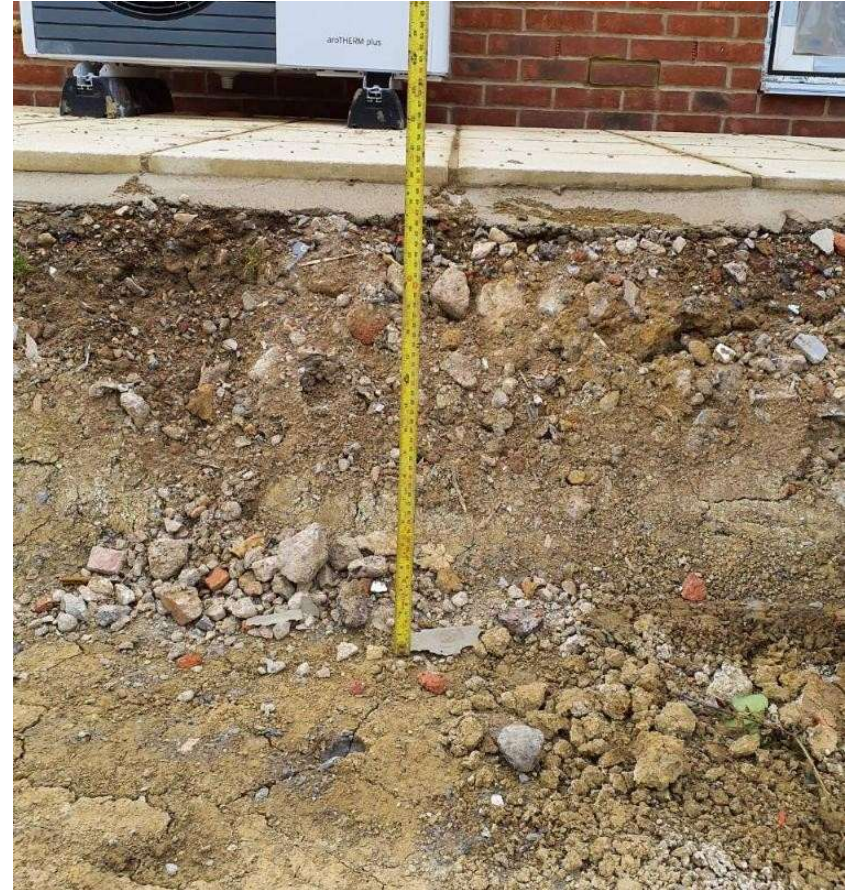
Tape measure showing reduction in formation level 400mm below final level in Plot 12
