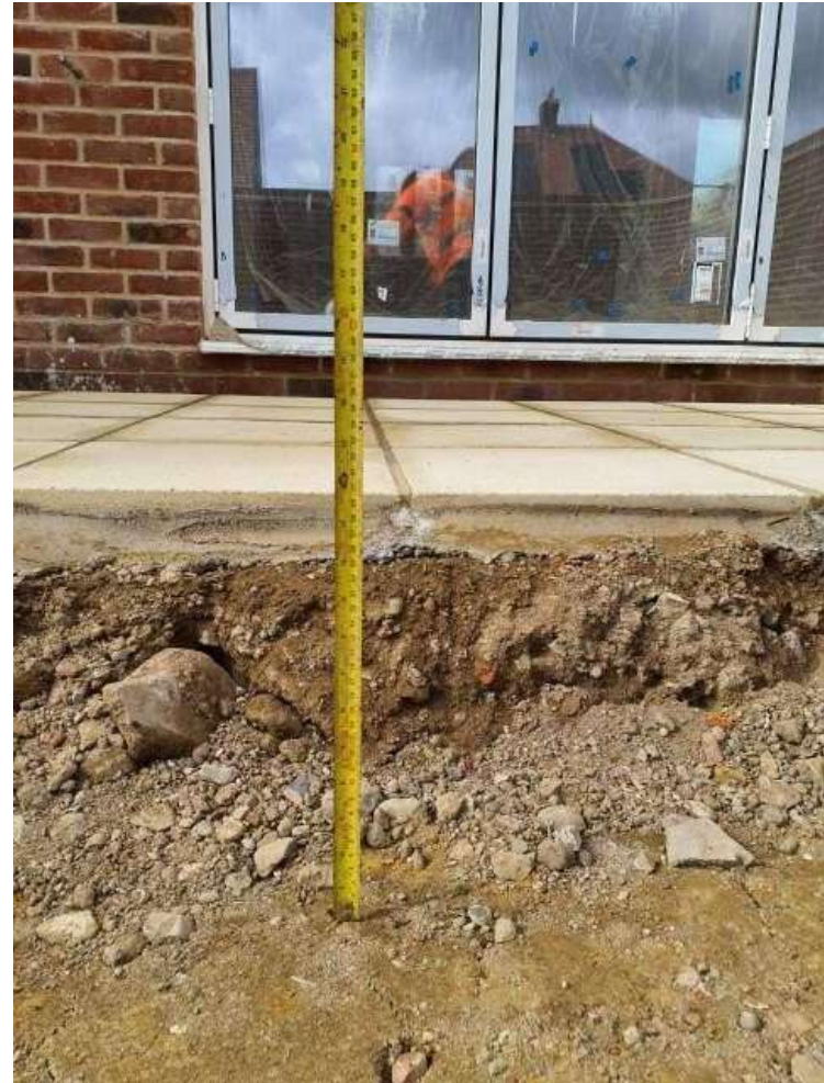
Depth from finished level to formation level in Plot 7
