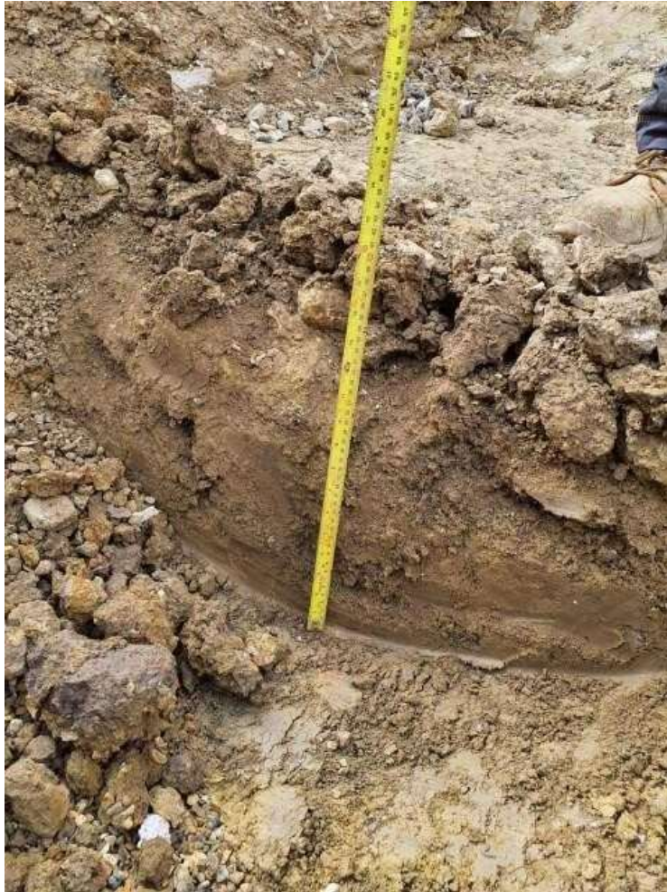
Pit excavated into formation level of Plot 7
