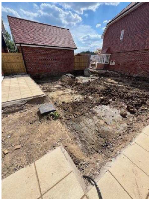
View of Plot 2 following removal of made ground in top 600mm (photograph provided by client)
