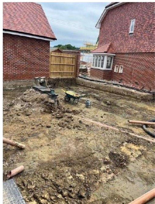
View of Plot 2 following removal of made ground in top 600mm (photograph provided by client)
