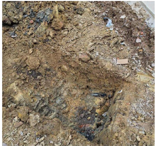
Inspection pit in Plot 2 indicating presence of made ground soils
