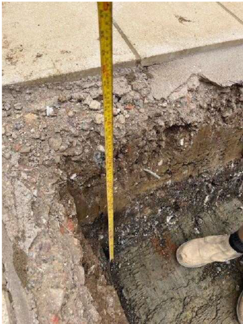
Tape measure comparing formation level from finished level, indicating formation level ~ 800 mm below finished level (photo provided by client)
