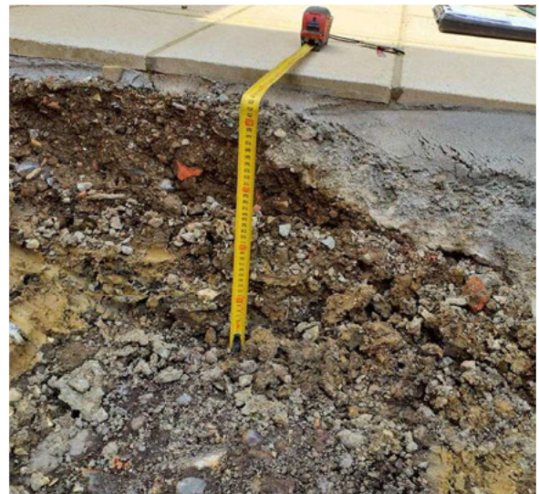
Tape measure showing comparison of finished level to formation level at time of visit, approximately 430mm.
