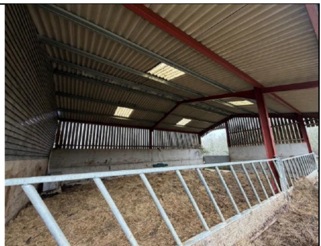
Photograph 14: Open sided extension on the northern elevation.
