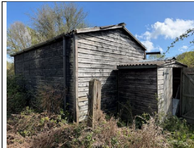
Photograph 21: Outbuilding and shed viewed from the northwest.
