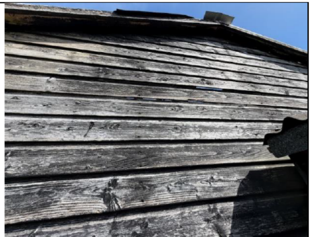
Photograph 22: Showing the single skin structure.
