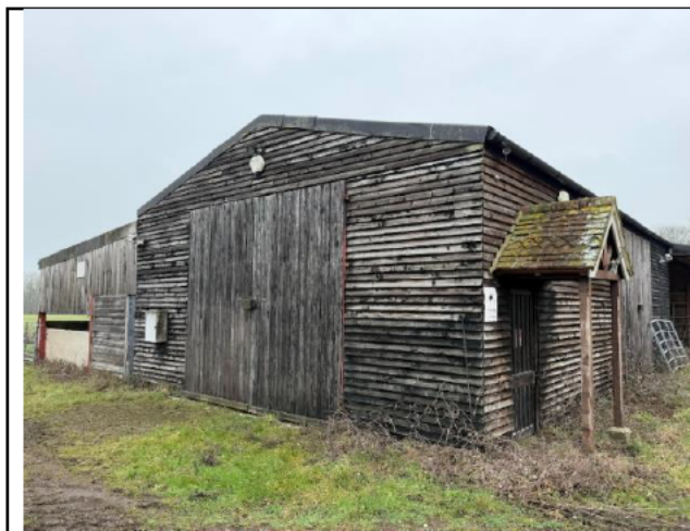
Photograph 13: Southern and eastern elevations of the agricultural building.
