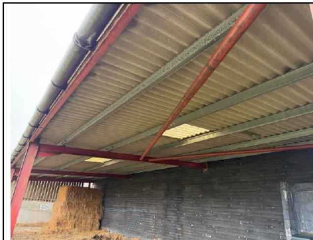
Photograph 15: Open sided extension on the western elevation.
