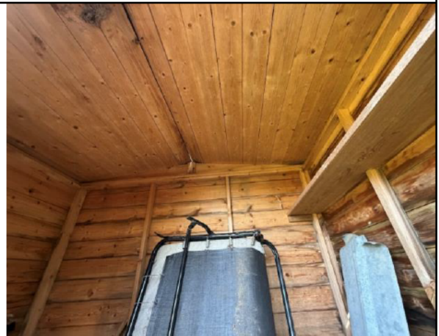
Photograph 24: Interior of the shed.
