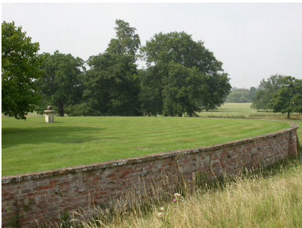
4. Ha-ha wall Brick and flint to match the building, or alternatively a rubble stone wall. Wall to be finished with a natural stone coping in a buff tone, cut to follow curved geometry.
