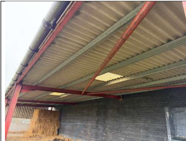
Photograph 15: Open sided extension on the western elevation.
