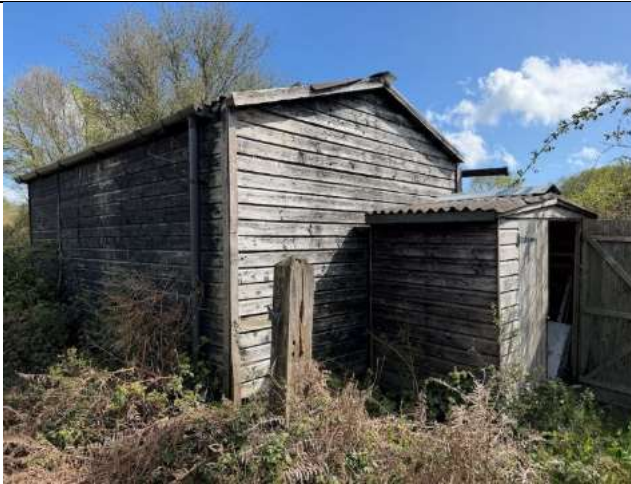
Photograph 21: Outbuilding and shed viewed from the northwest.
