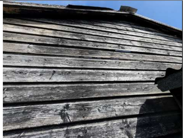
Photograph 22: Showing the single skin structure.
