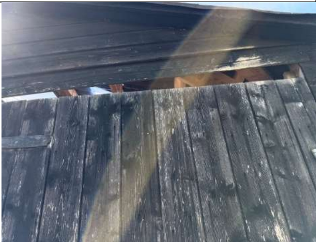
Photograph 23: Showing bright internal conditions.
