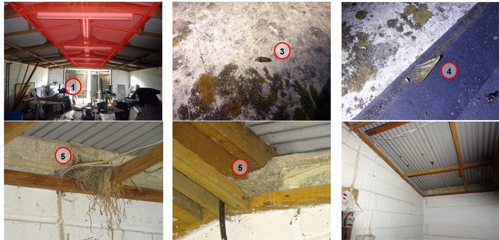
Building B1 — Internal Inspection, Section Two, Confirmed Roost
