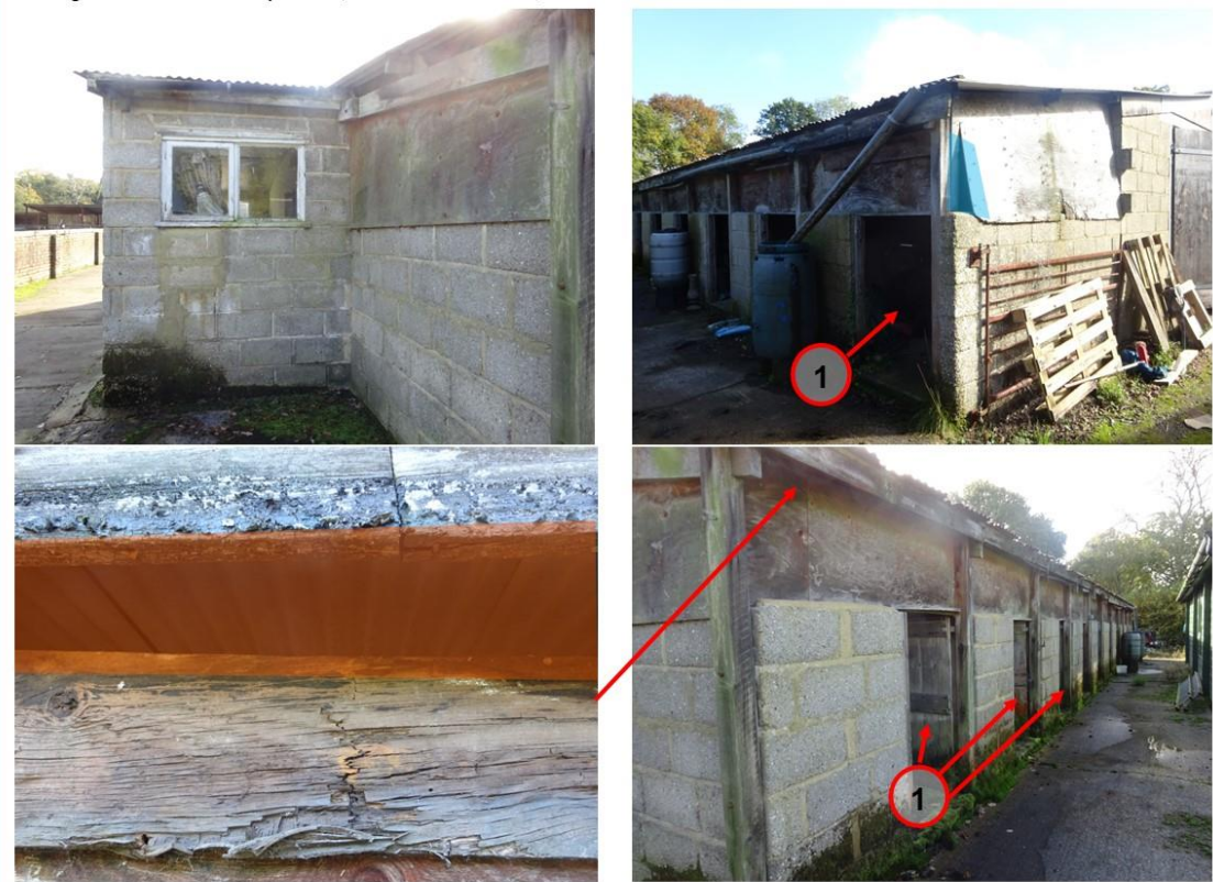
Building B1 — External Inspection, Western Elevation, Confirmed Roost
