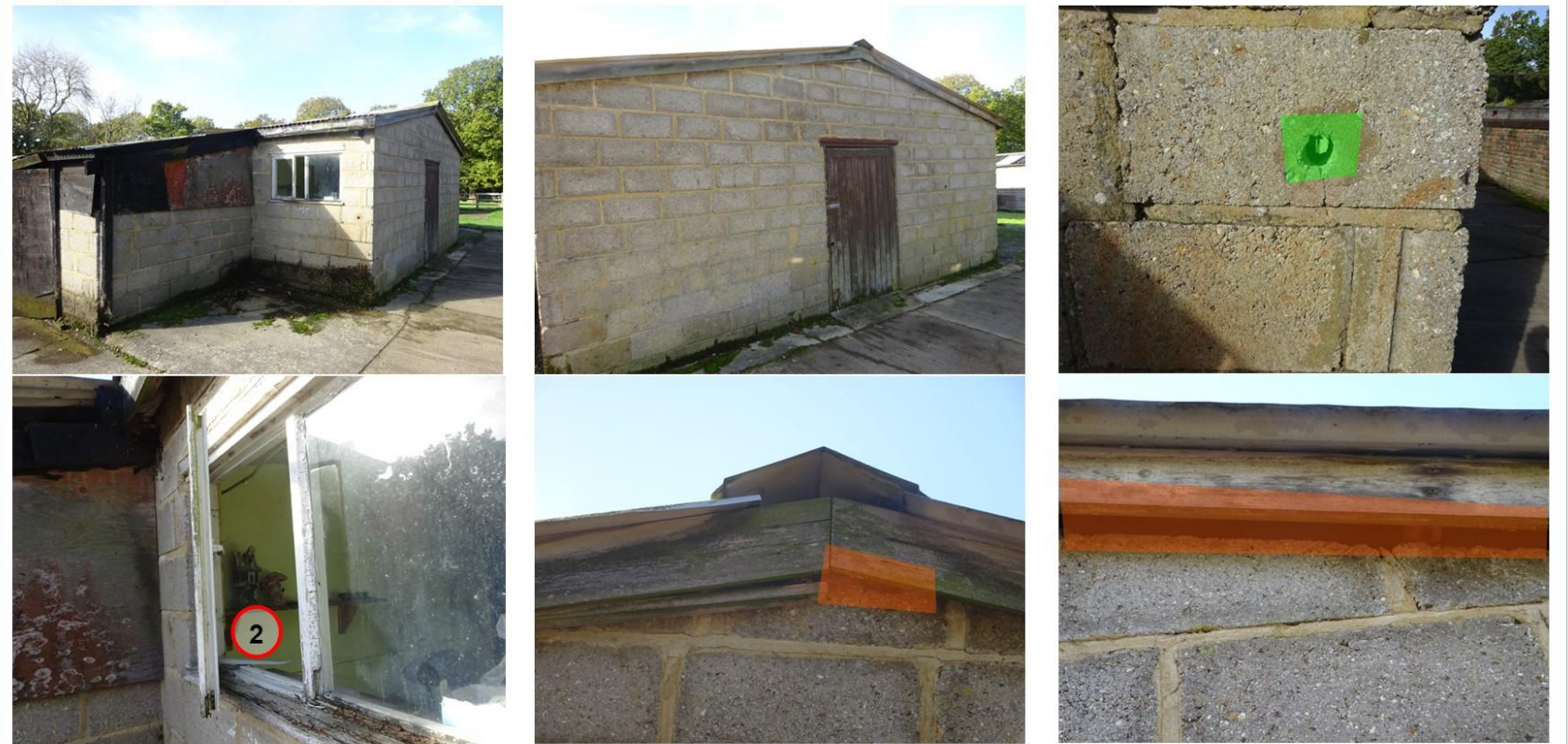
Building B1 — External Inspection, Northern Elevation, Confirmed Roost
