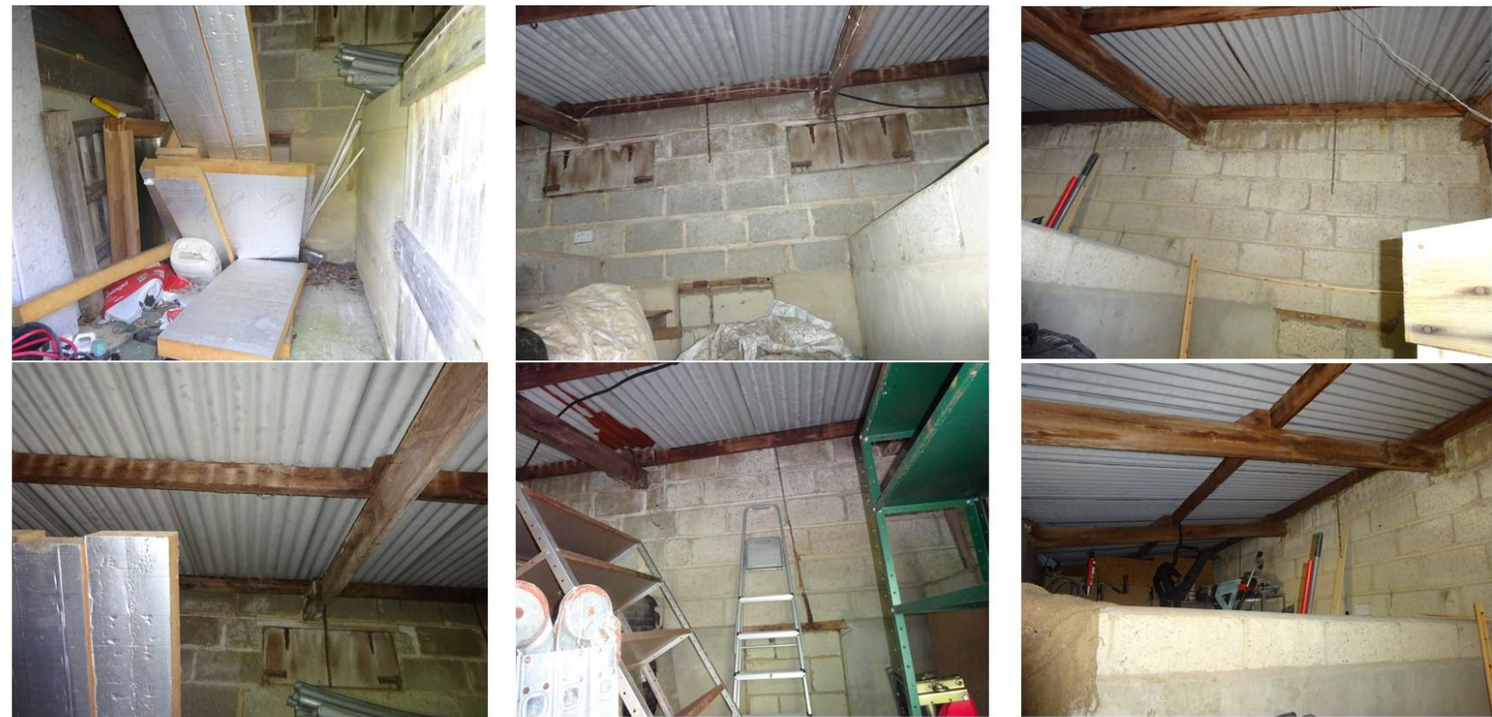
Building B1 — Internal Inspection, Western Stables, Confirmed Roost
