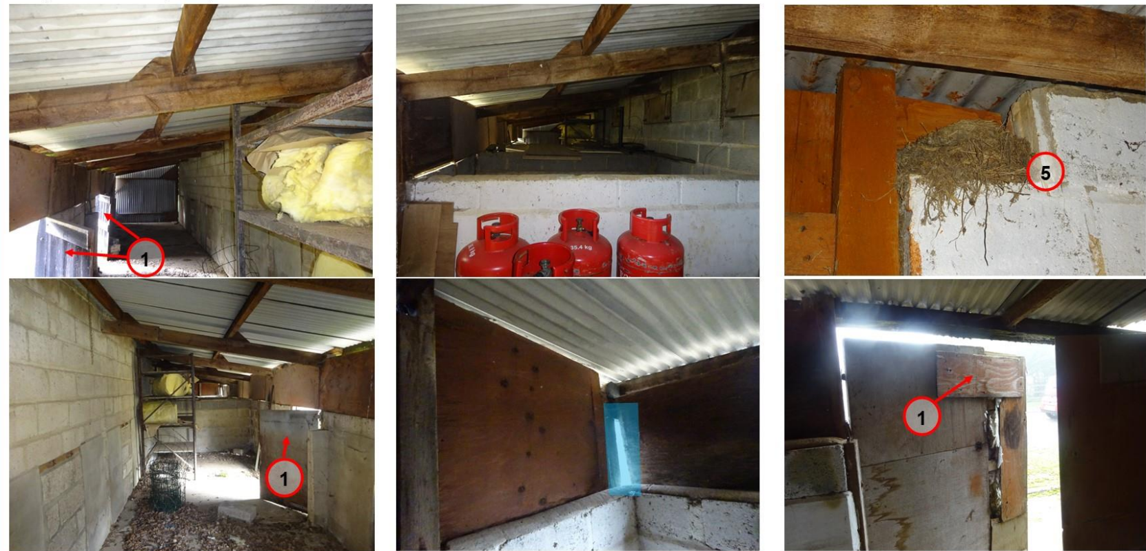
Building B1 — Internal Inspection, Eastern Stables, Confirmed Roost
