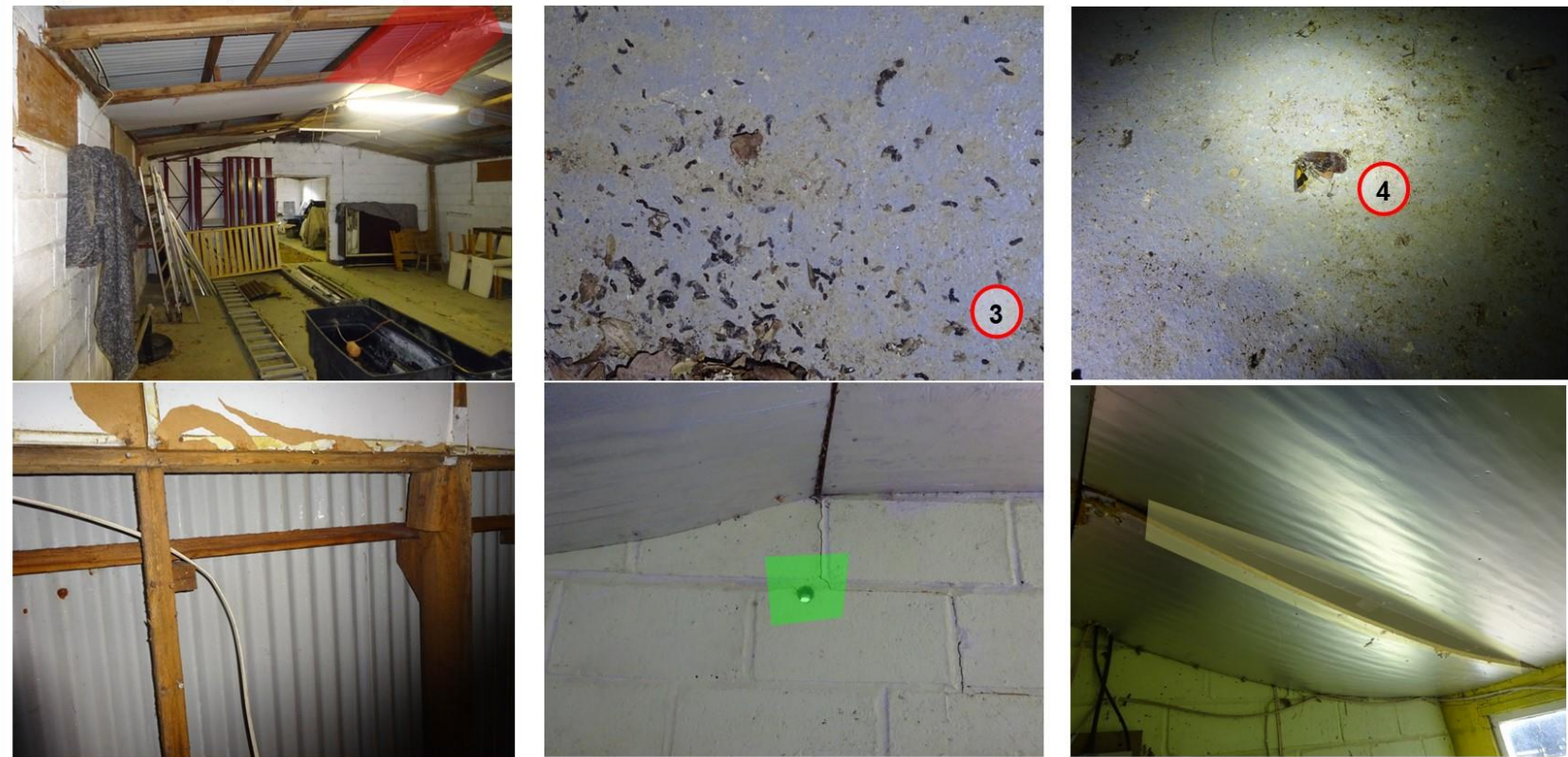
Building B1 — Internal Inspection, Section One, Confirmed Roost
