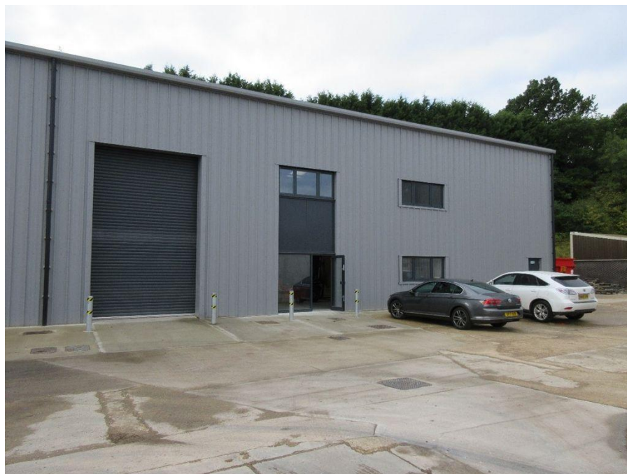
Building 3 - West Unit
