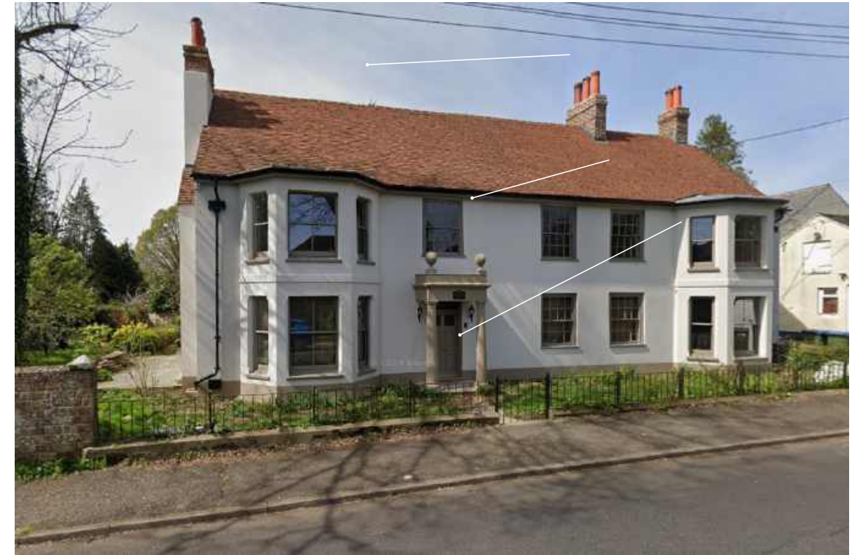
Grade II listed Wood Grange
