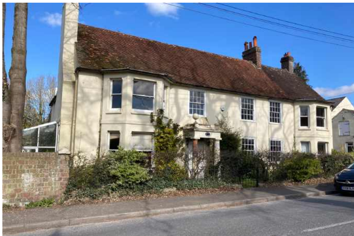
East elevation of Wood Grange, prior to removal of 20th century conservatory to the south elevation
