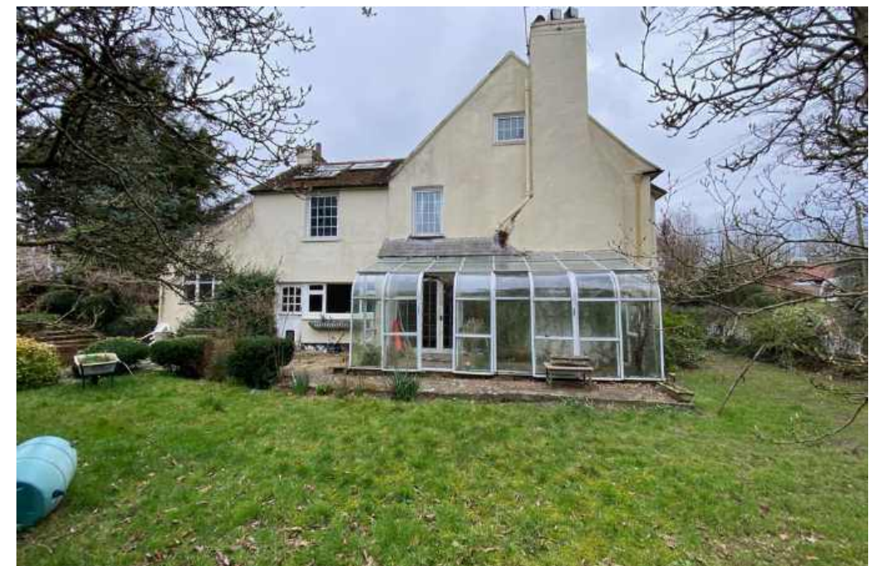
South elevation of Wood Grange, prior to removal of 20th century conservatory
