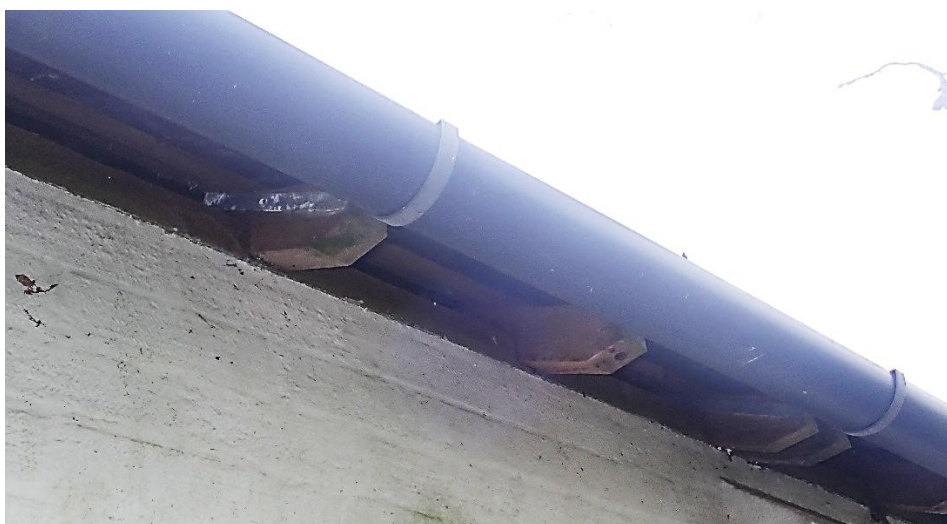
Fig. 7 – View to eaves of building
