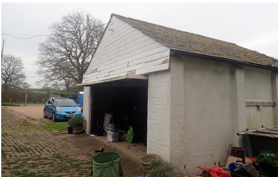
Fig. 6 – The garage, viewed from the south-west
