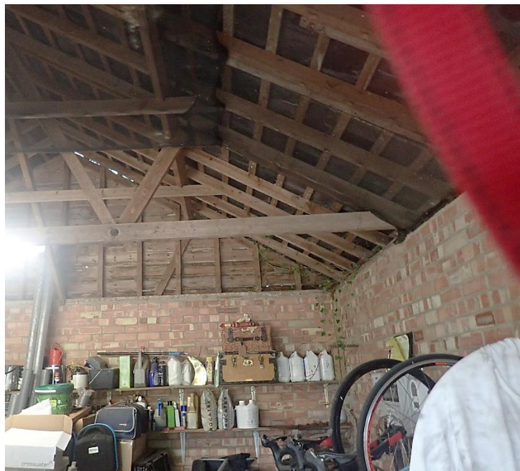
Fig. 9 – Interior view of garage
