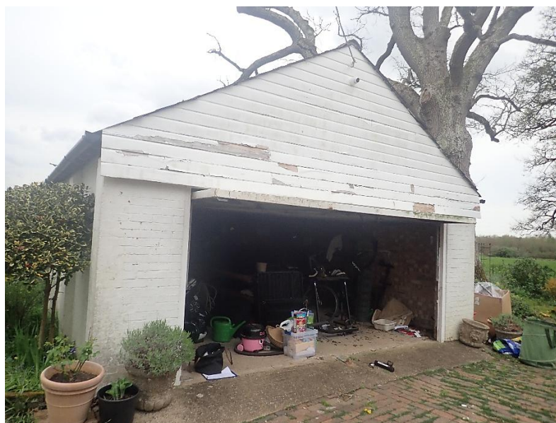
Fig. 5 – Entrance to garage (west side), with timber cladding above
