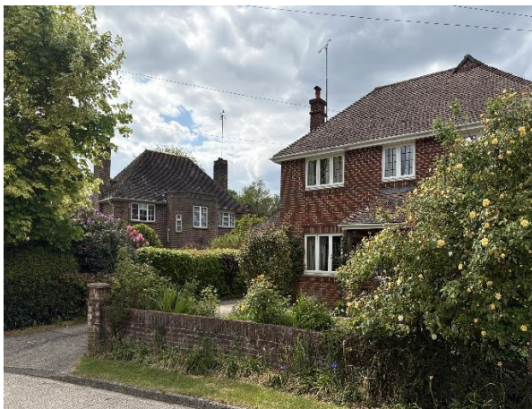
Penn Cottage with Sandycroft in background
