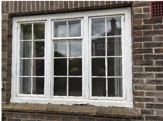
Examples of poor condition of the single glazing
