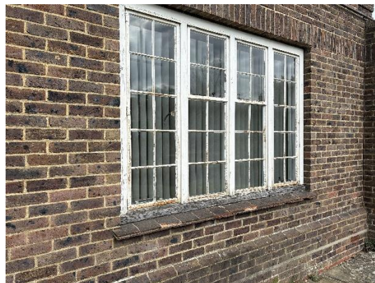
Examples of poor condition of the single glazing
