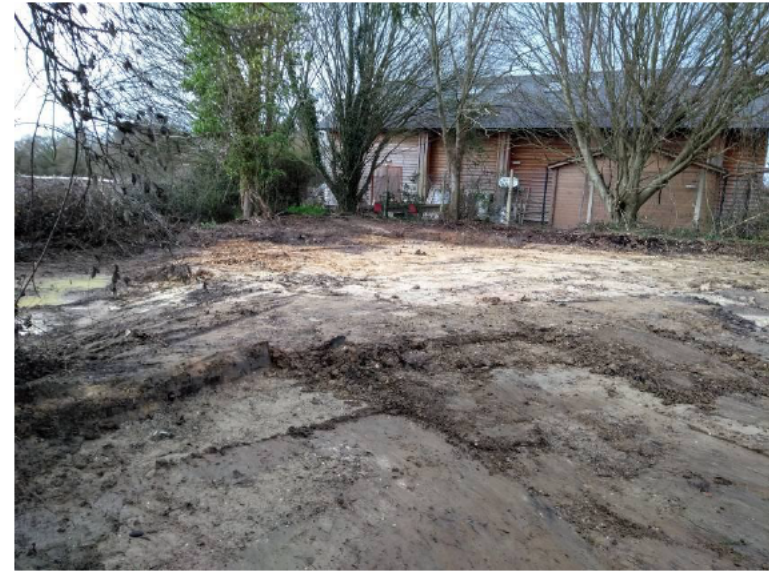
Plate 2: SW corner of Plots 1 & 2 following the removal of the residual Made Ground
