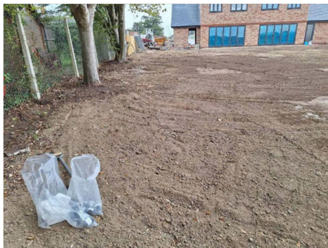
Plate 6: Southern part of Plot 1 completed (STL 01.10.2025).
