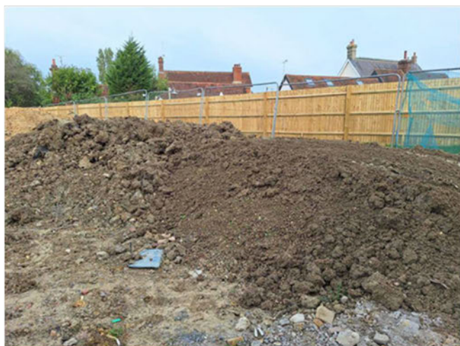
Plate 9: Stockpile TS1 in plots 9 & 10 (STL 01.10.2025)
