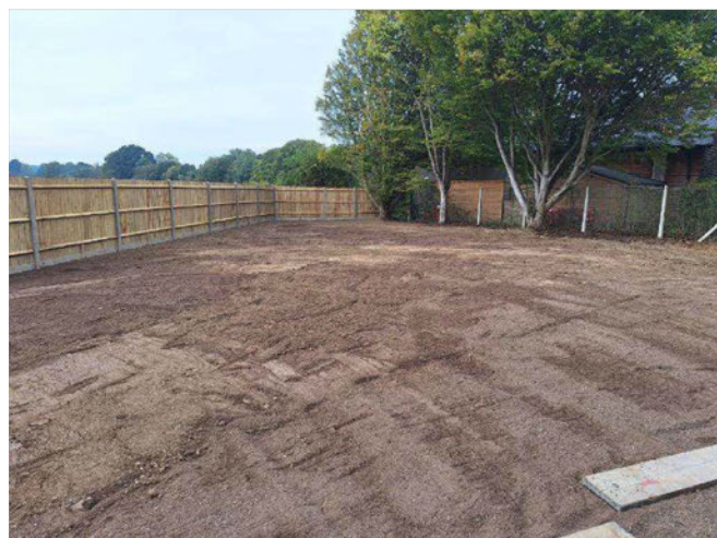
Plate 8: Plot 1 & 2 completed (STL 01.10.2025).
