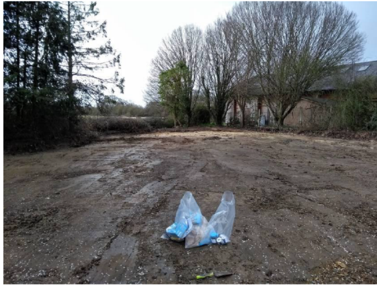
Plate 1: Looking SW across plots 1 and 2 following the removal of the residual Made Ground
