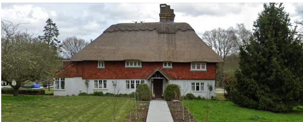
Figure 2 - External View of Shuckers Farmhouse (Google Maps, 2025)
