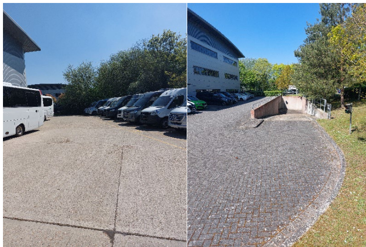
Photograph Nos: 5 and 6 – Developed land; sealed surface within the site, including the southern car parking area, the existing building and the entrance to the underground car park.
