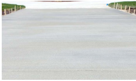
Concrete paving - South Car parking Areas
