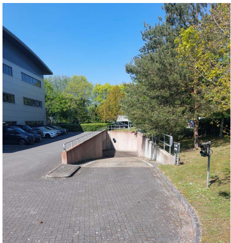
Photograph C - Sloping access leading to the underground car park.
