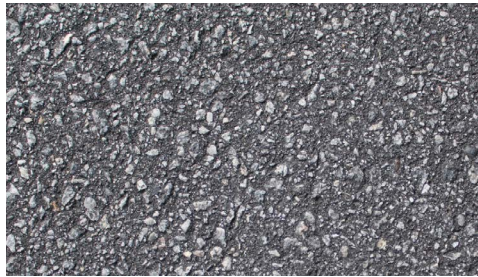
Mid Grey Asphalt - Pedestrian Access
