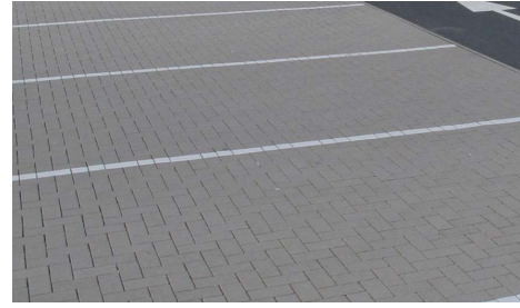
Block paving - North Car Parking Areas - Grey
