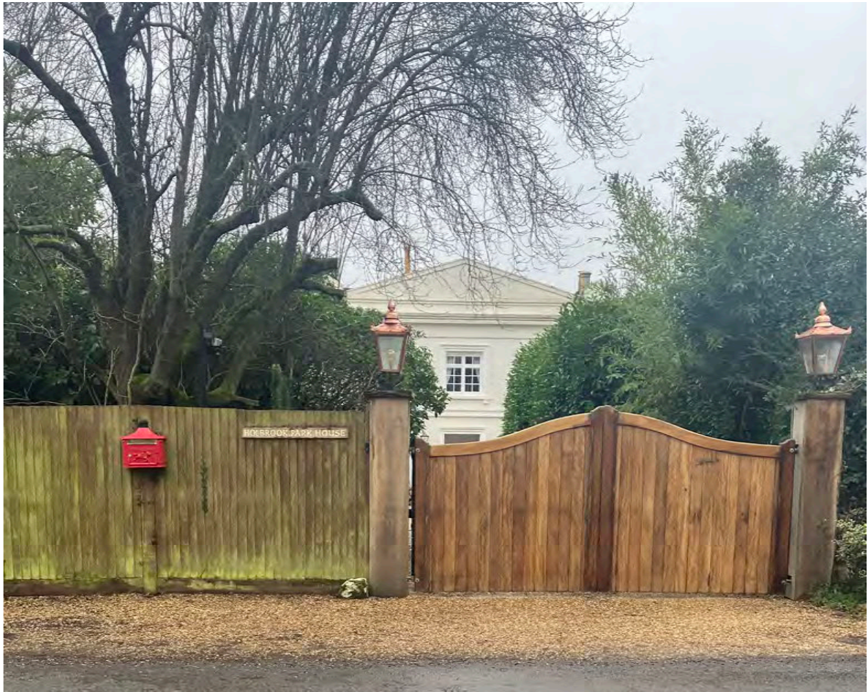
Plate 14: View of the Grade II listed Holbrook Park House from Old Holbrook
