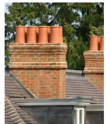
Sussex Stack Chimney
