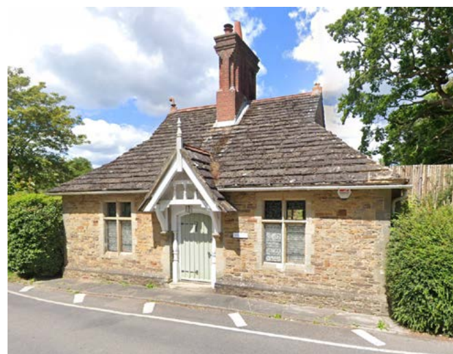
07. Listing Name: Old Lodge to North East of Christ's Hospital List Entry No: 1027033 Grade: II Date Listed: 28 November 1980
