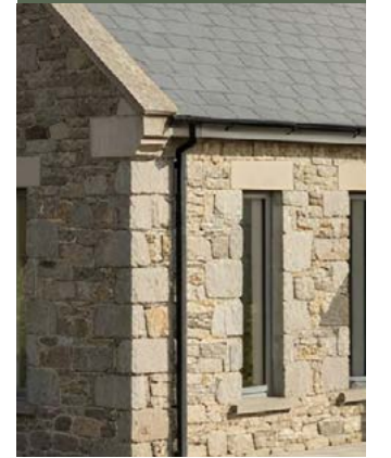
Stone Cornice and Quoin Detail
