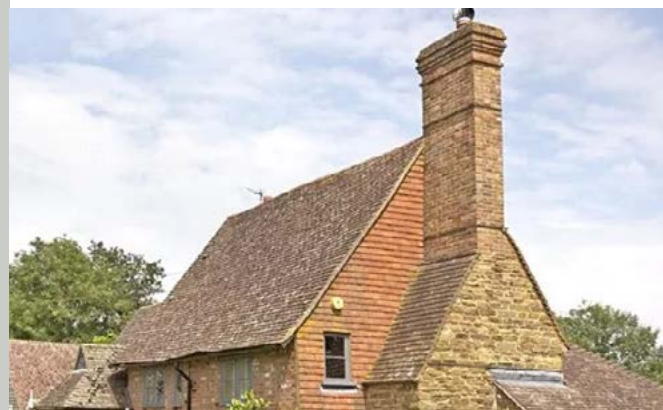
Gable and 'Sussex Stack' Chimney
