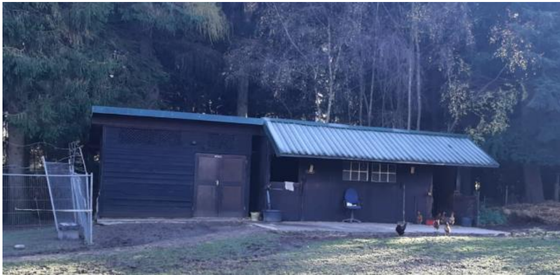
Existing Building December 2025
