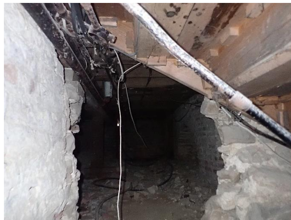
Fig. 13 - View into unconverted section
