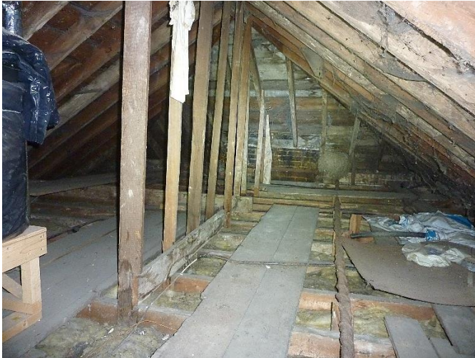
Fig. 7 - Roof Void with timber sarking beneath slates
