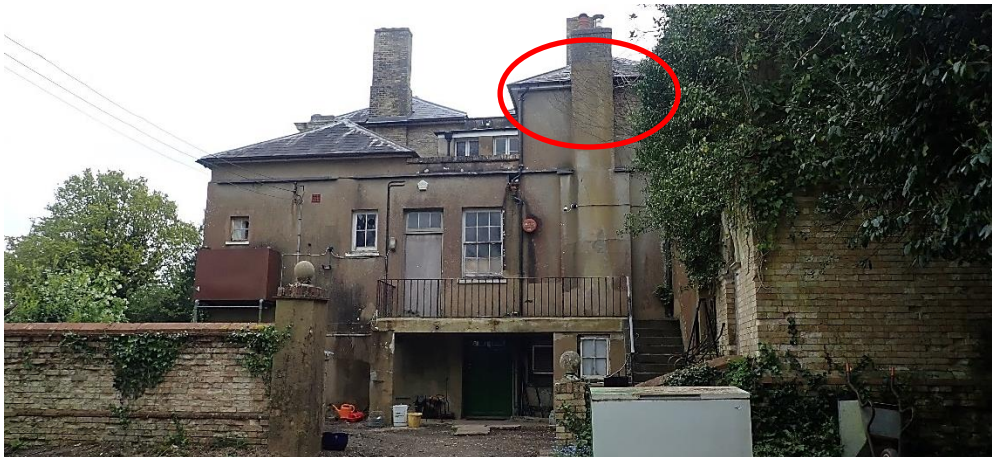
Fig. 4 – View of west side house, showing inaccessible area of roof (circled)
