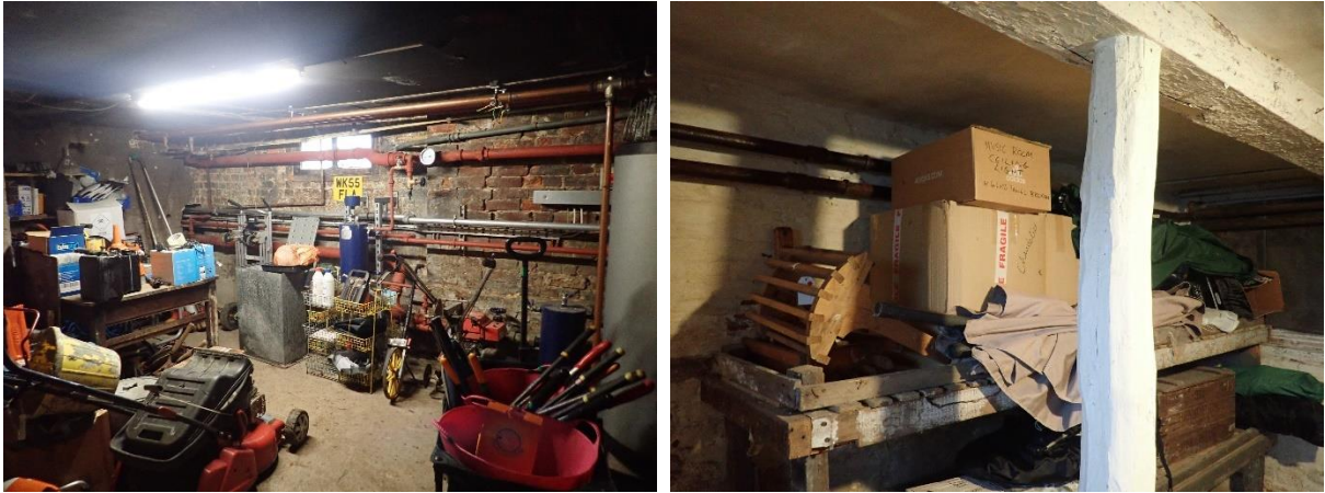
Figs. 11/12 - Views of basement rooms
