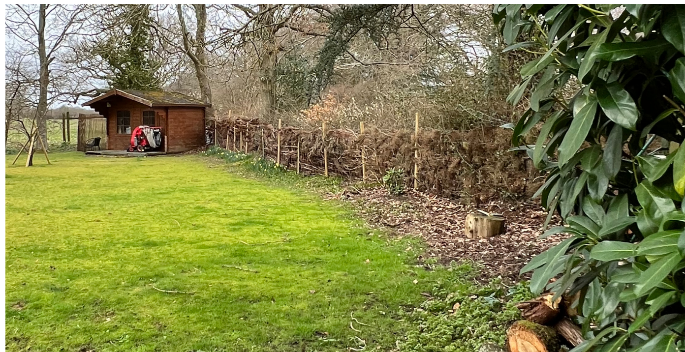
Area of fence to be replaced
