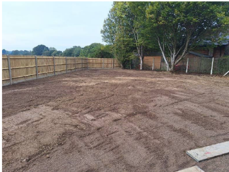
Plate 3: Plot 2 (foreground) and Plot 1 completed.
