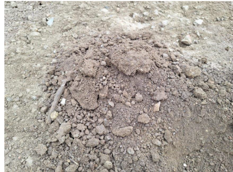
Plate 4: Site won soils placed in Plot 2.
