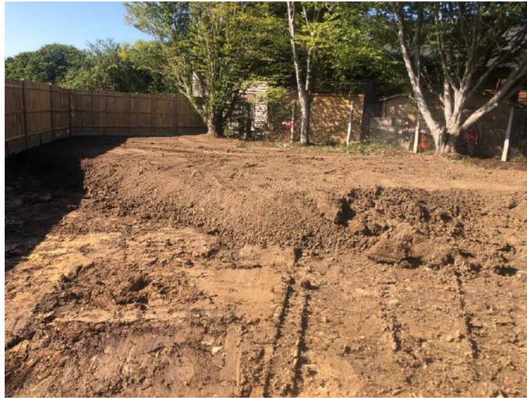
Plate 1: Photograph provided from site showing the placement of topsoil.
