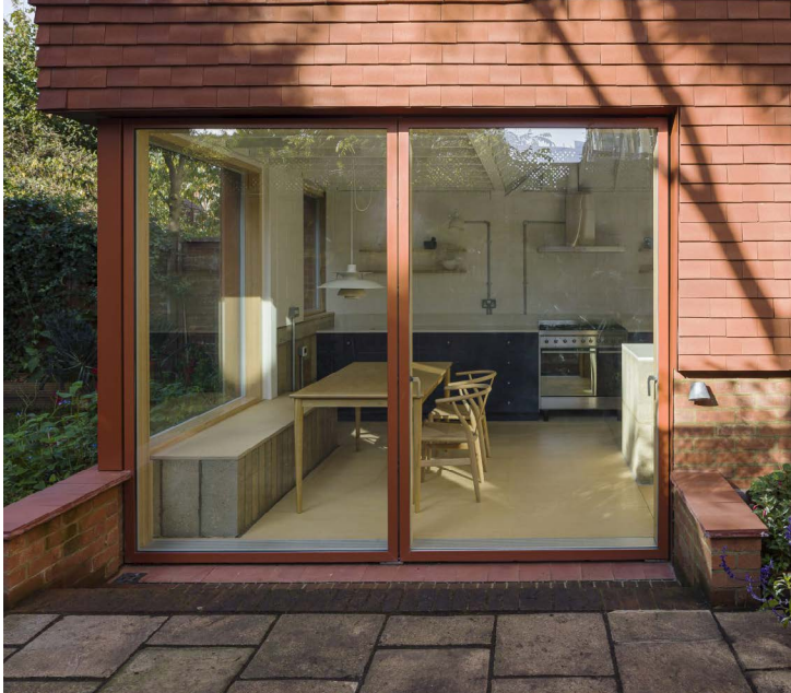
Corner glazing with red tiles over.
