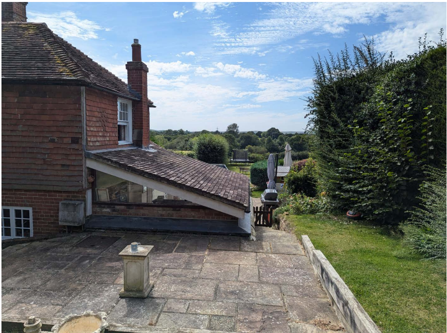
Later addition western extension and single storey extension
