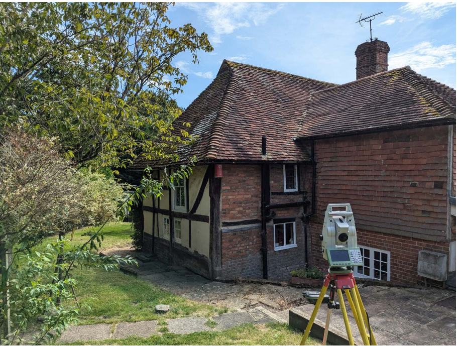
North facing elevation showing later addition extension and original timber frame house.
