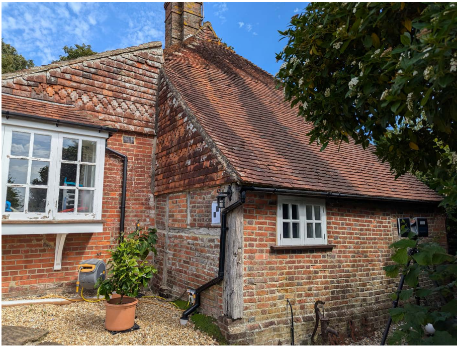
South West Elevation, Lounge Bay Window and cat slide roof
