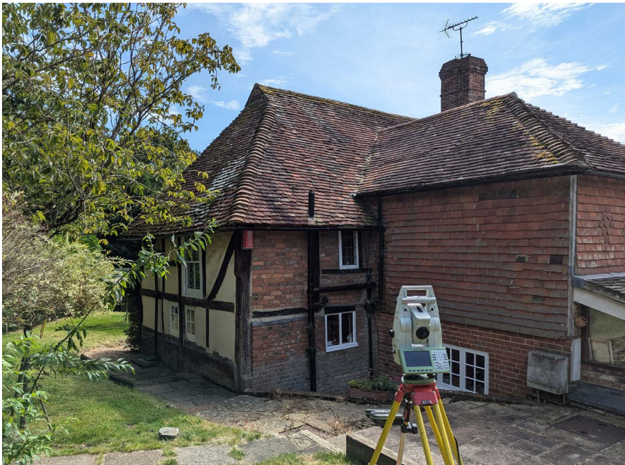
North West Facing Elevation of original house.
