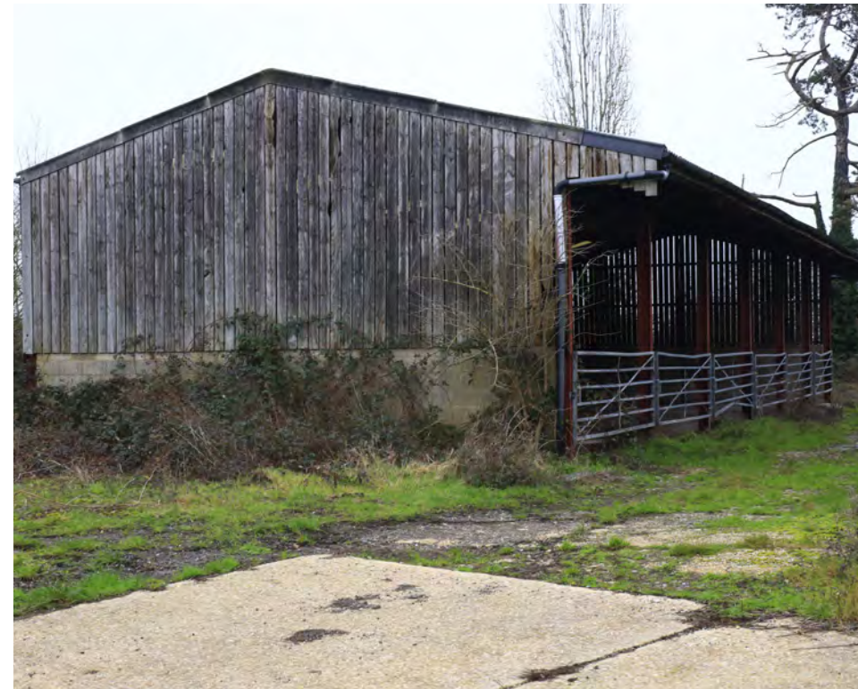
11: Building B2 [Northern Edge]
