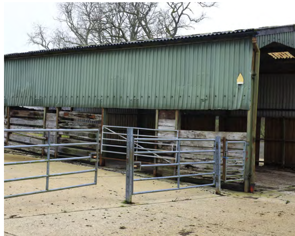
05: Building B7 & Associated Concrete Hardstanding
