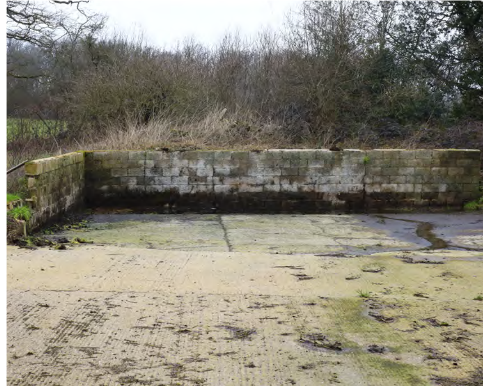
08: Concrete Retaining Structure [Western Edge]
