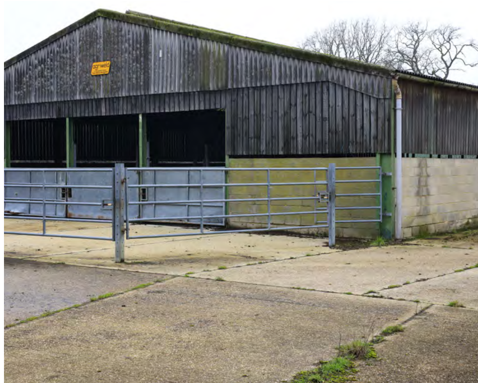
04: Building B3 & Associated Concrete Hardstanding
