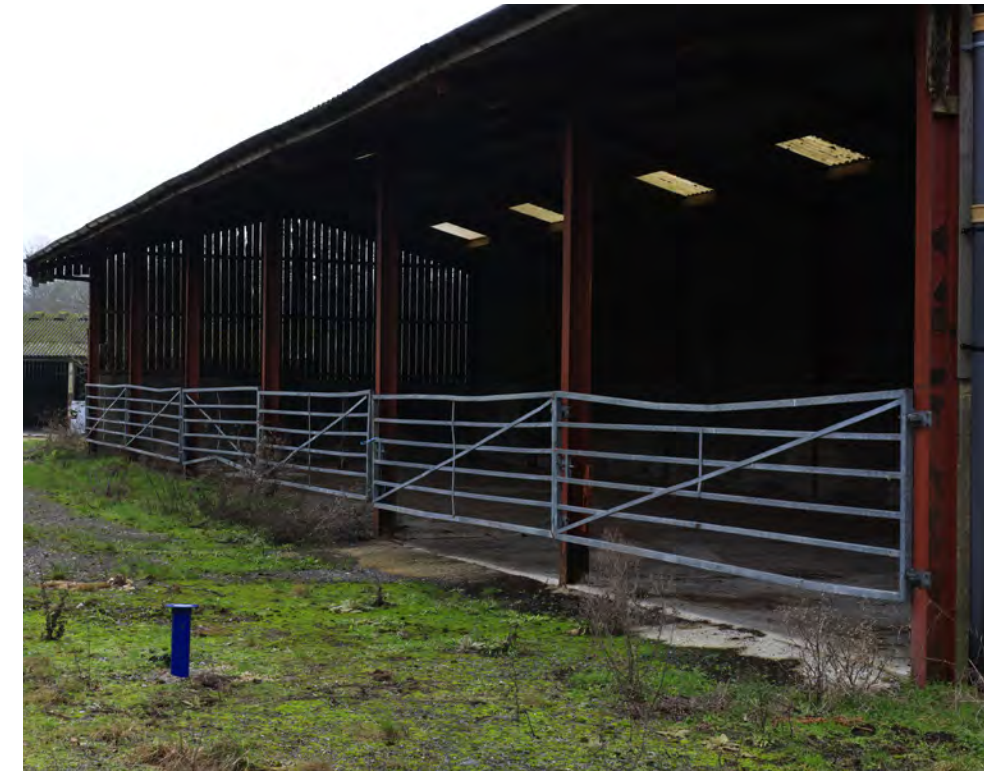
12: Building B2 [Northern Edge] Looking West
