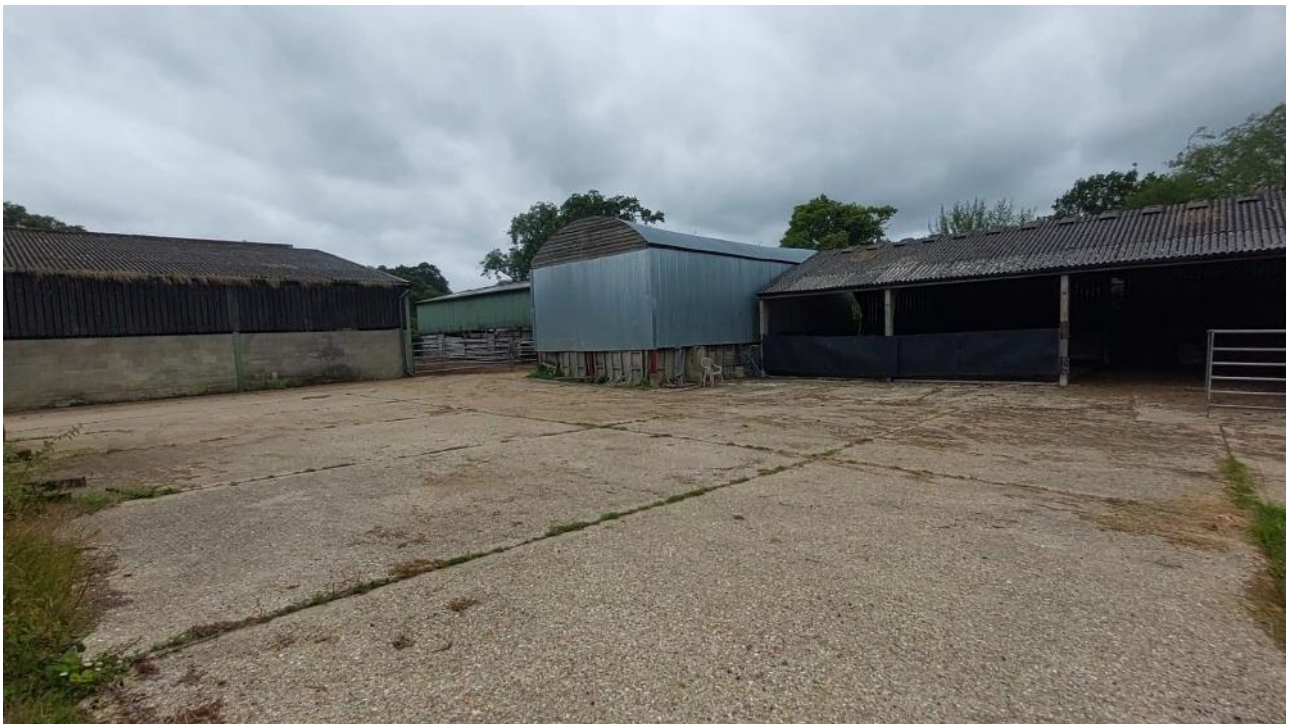
Image 10 – the hardstanding land located in the centre of the site.
