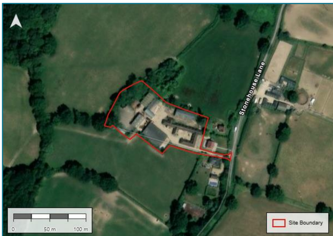
Figure 2.1 – Aerial View of Existing Site
