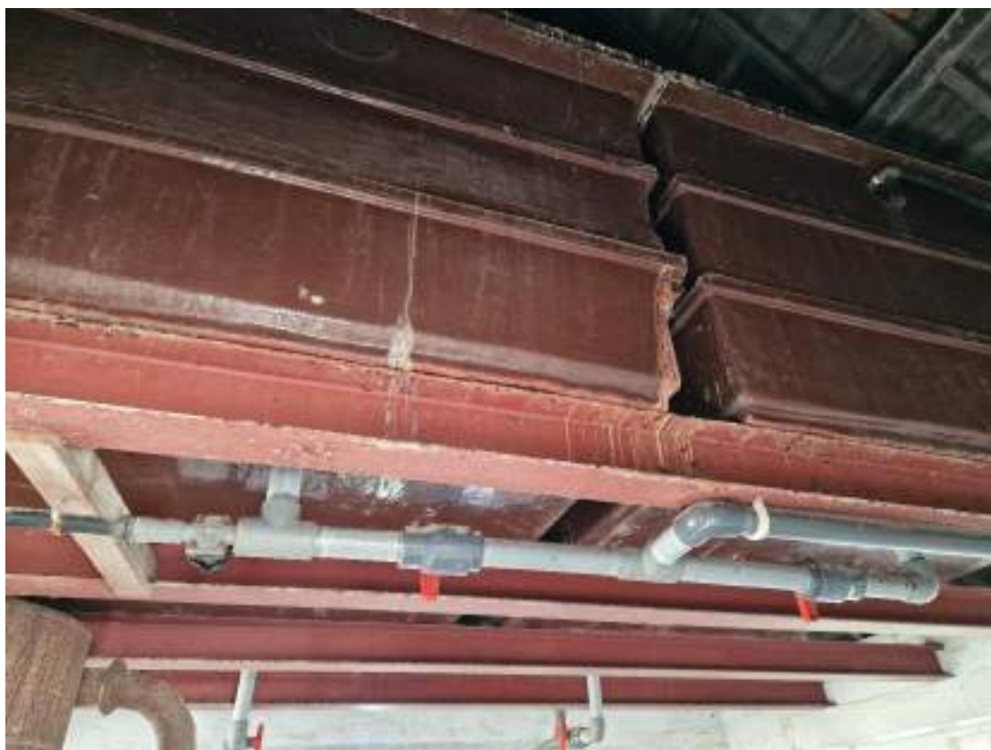
B1 stored overhead tanks
