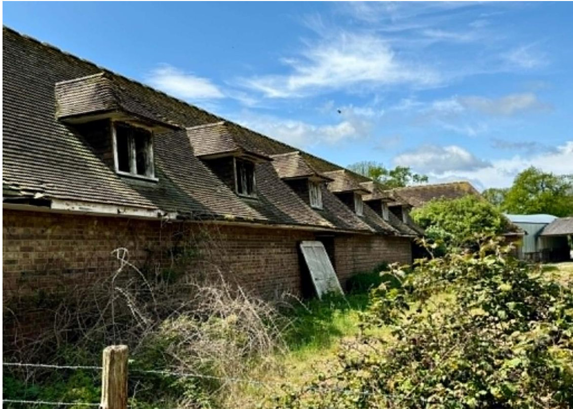
Fig 7: The north elevation of the stable block showing a line of dormer windows and coursed brickwork. The building, which has never been altered, will be restored and given a sustainable residential use.
