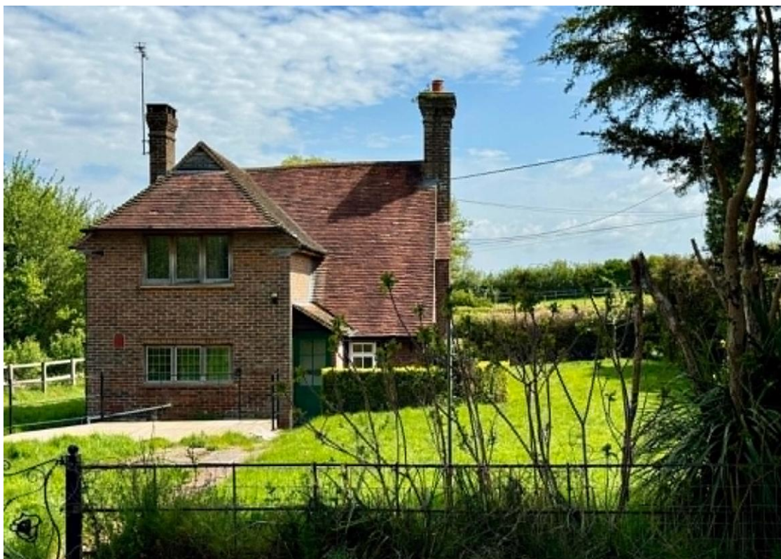
Fig 10: Little Patches as seen from the proposed site towards its rear (west) elevation. This contains a modern two storey extension, finished in a matching style, that is of least significance to the listed building.
