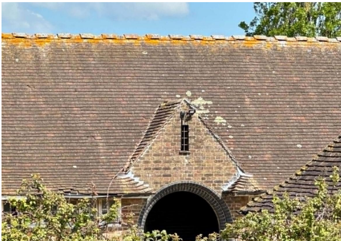
Fig 8: The inner courtyard of the stable block contains some fine detailing including the use of grey headed brick and through archways. These architectural features add to the merit of the historic building.
