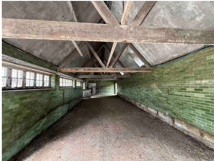
Internal View of Existing Stables
