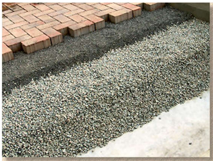
Figure 9: Typical permeable paving solution
