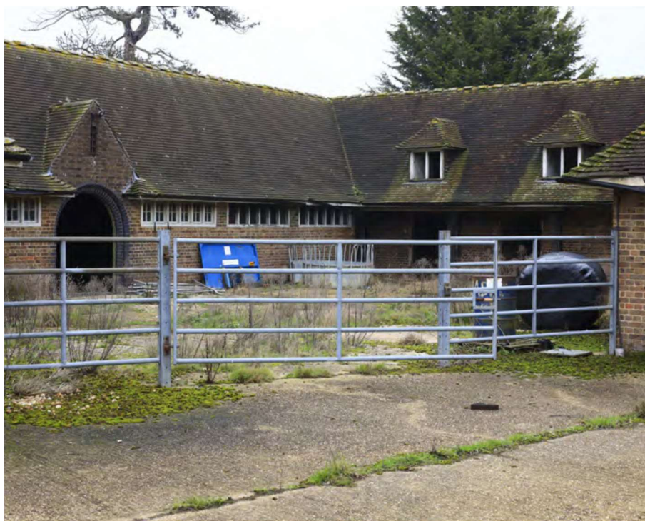
Figure 10: Stables to be converted and associated courtyard
