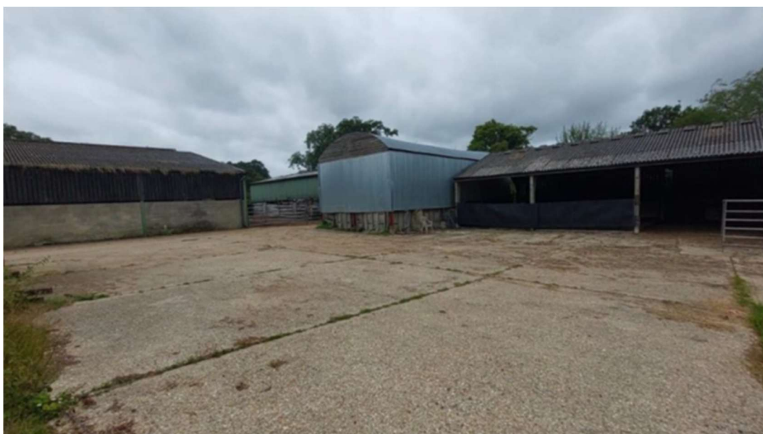
Figure 11: Main courtyard area of hardstanding and associated buildings
