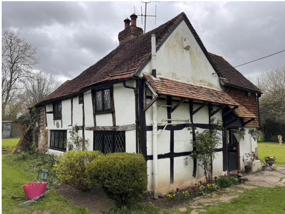
Photo (i) – entrance and front elevation
