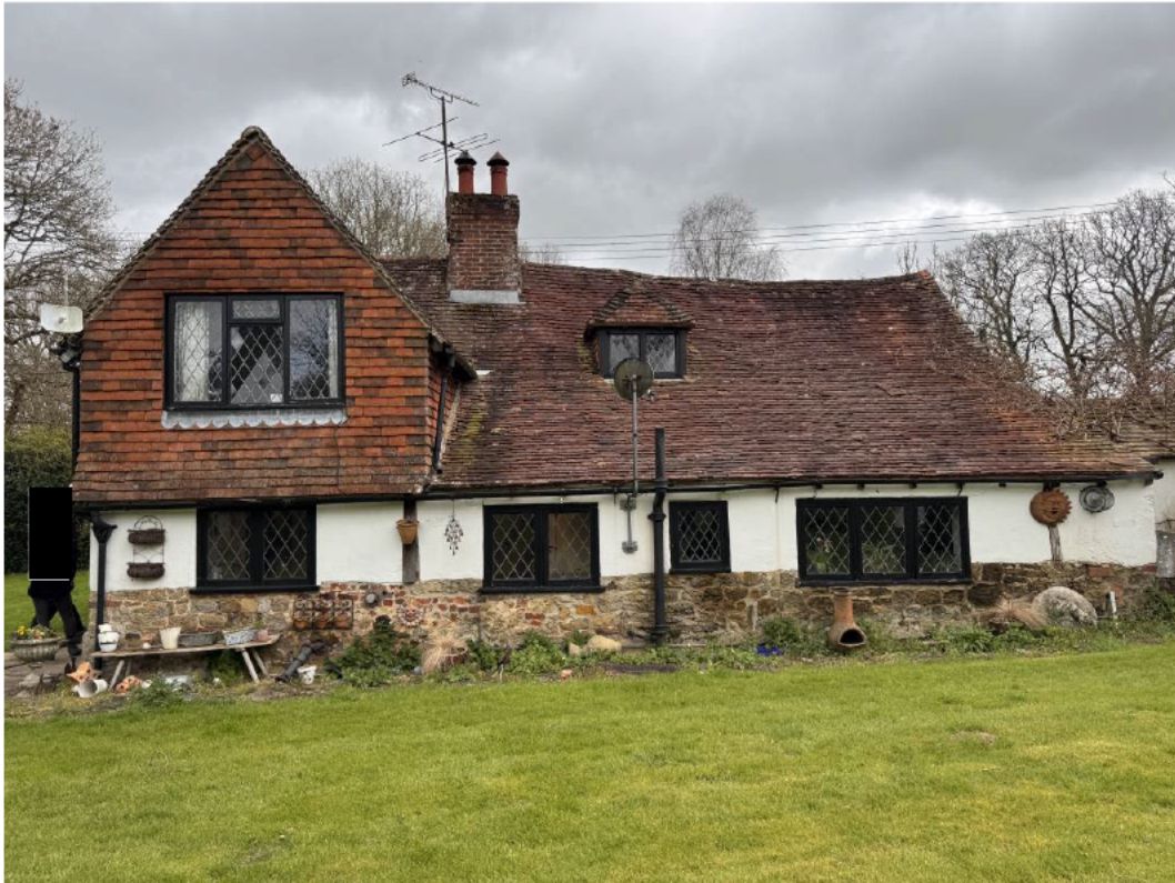
Photo (ii) – rear elevation
