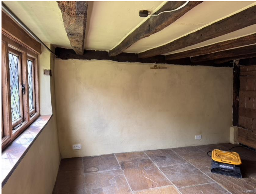
Photo (v) – typical plastered wall
