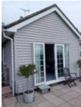
V2 B1-3 surveyor photo
