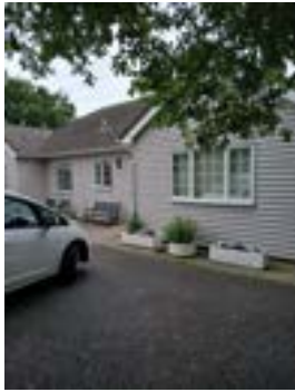
V2 B1-4 surveyor photo
