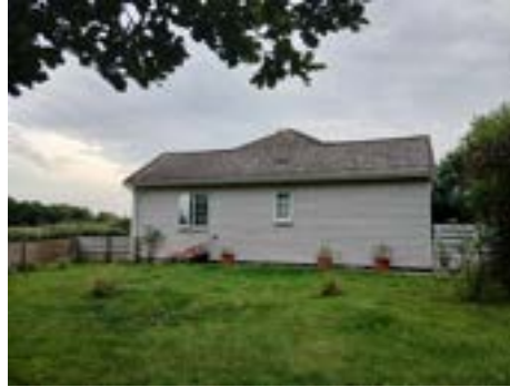
V2 B1-1 surveyor photo
