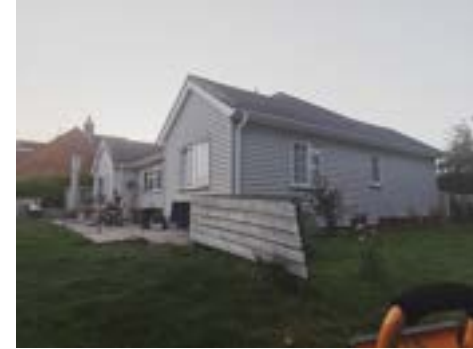
V1 B1-2 surveyor photo
