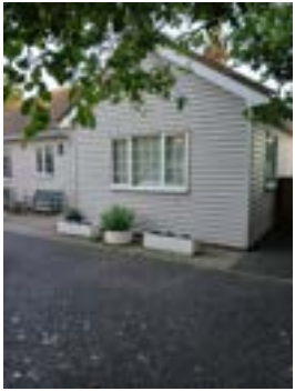
V1 B1-4 surveyor photo
