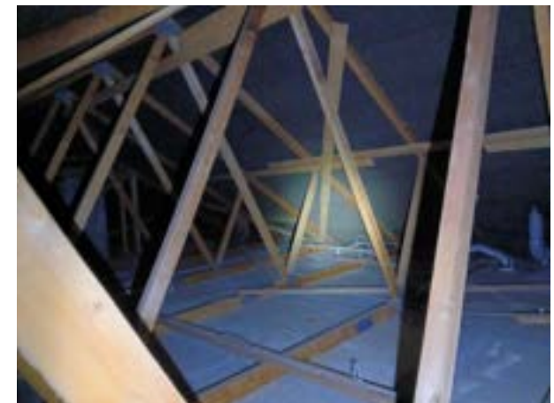
Figure 1b: Internal roof void of building B1 during the updated internal inspection
