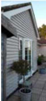
V1 B1-3 surveyor photo
