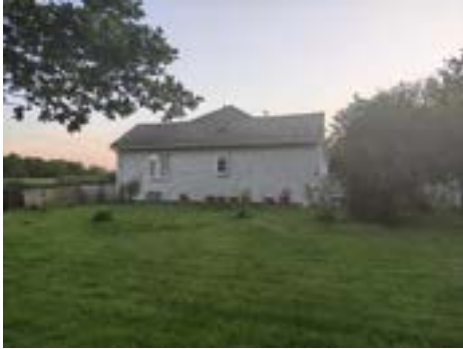
V1 B1-1 surveyor photo
