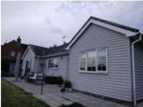
V2 B1-2 surveyor photo
