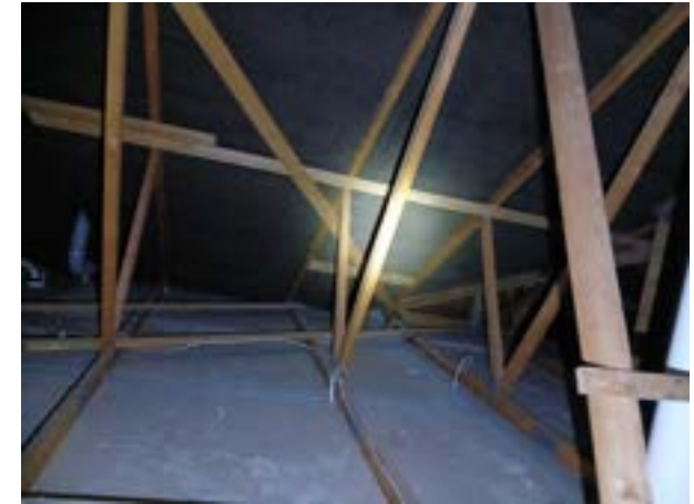
Figure 1a: Internal roof void of building B1 during the updated internal inspection
