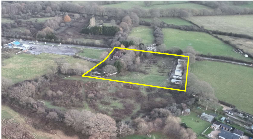
Fig. 4 – Aerial photograph Character Area 2 (CA2)
