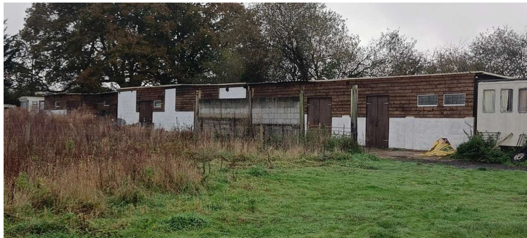
Fig. 5 – Farm/barn buildings on southwest boundary of CA2
