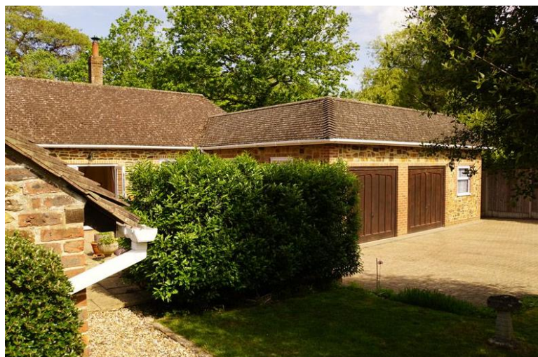
Figure 5 – Photographs of rear extension
