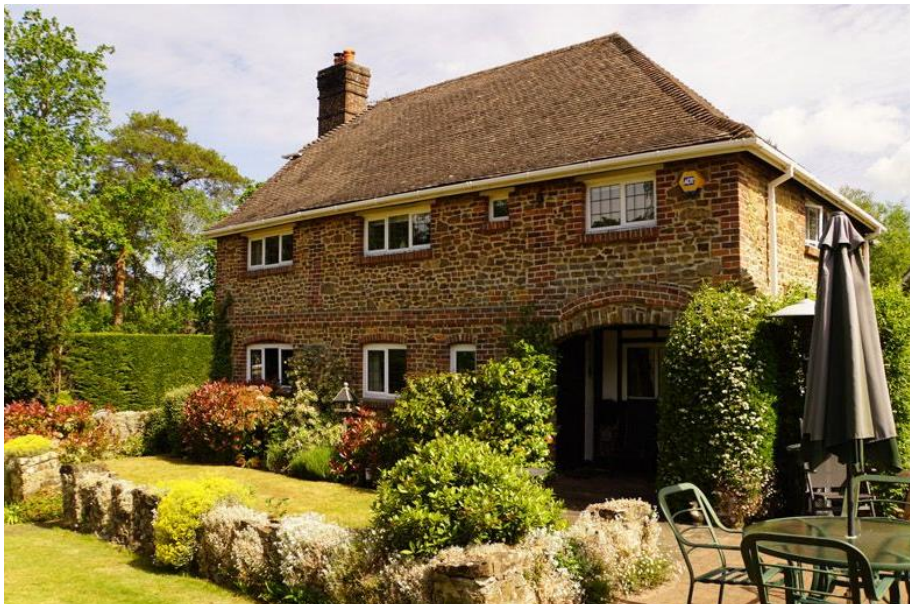
Figure 4 – Front elevation photograph of the application property
