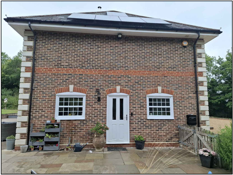
EXISTING SIDE VIEW - 2
