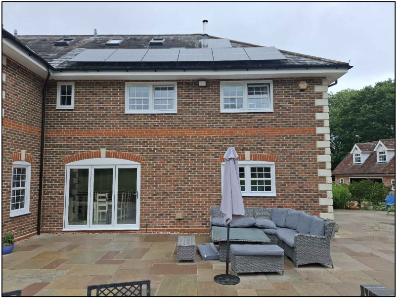
PART EXISTING REAR VIEW - 3
