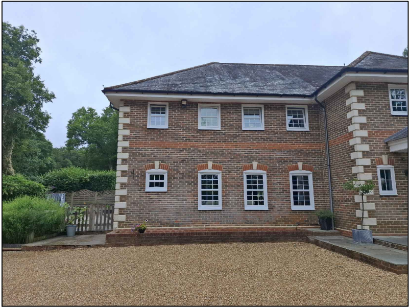
PART EXISTING FRONT VIEW - 1
