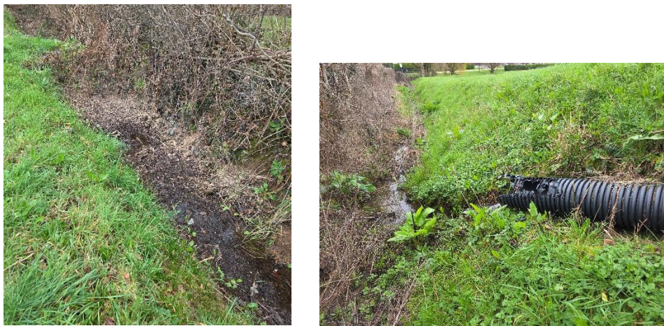
Figure 2-5 Diversion feature within on-site ditch (left) and outlet of diversion pipe (right)
